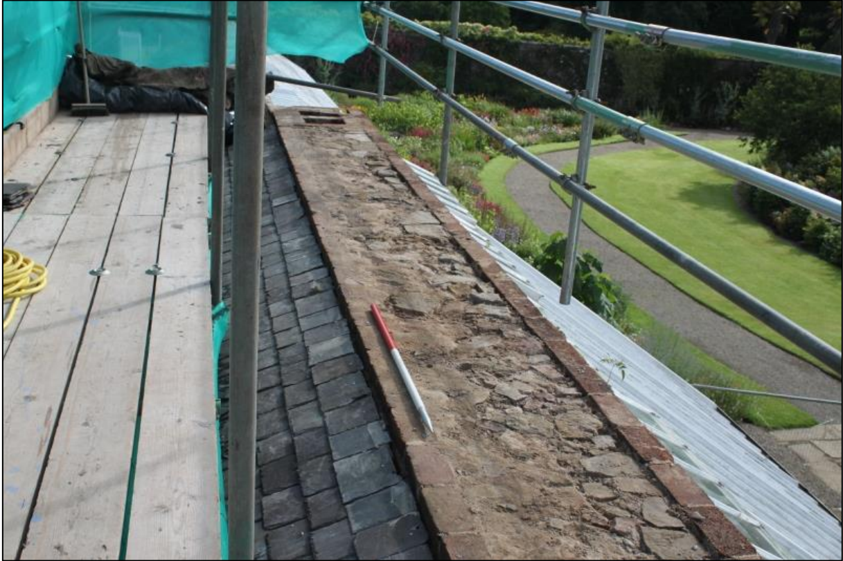
Figure 4a: Consolidated area at NE end of Spine Wall (0-10m SW of NE end)
