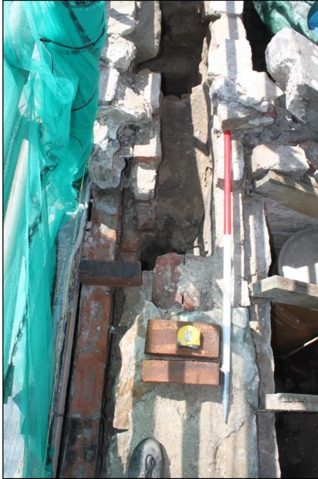
Figure 6a: Flues [013] (front) and [017] (rear), with change in wall configuration evident
