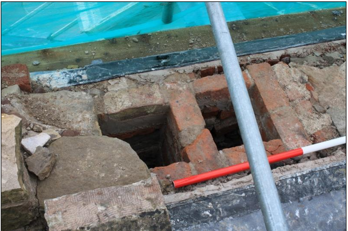
Figure 6b: Flues [022] and [024], handmade brick lining in upper courses
