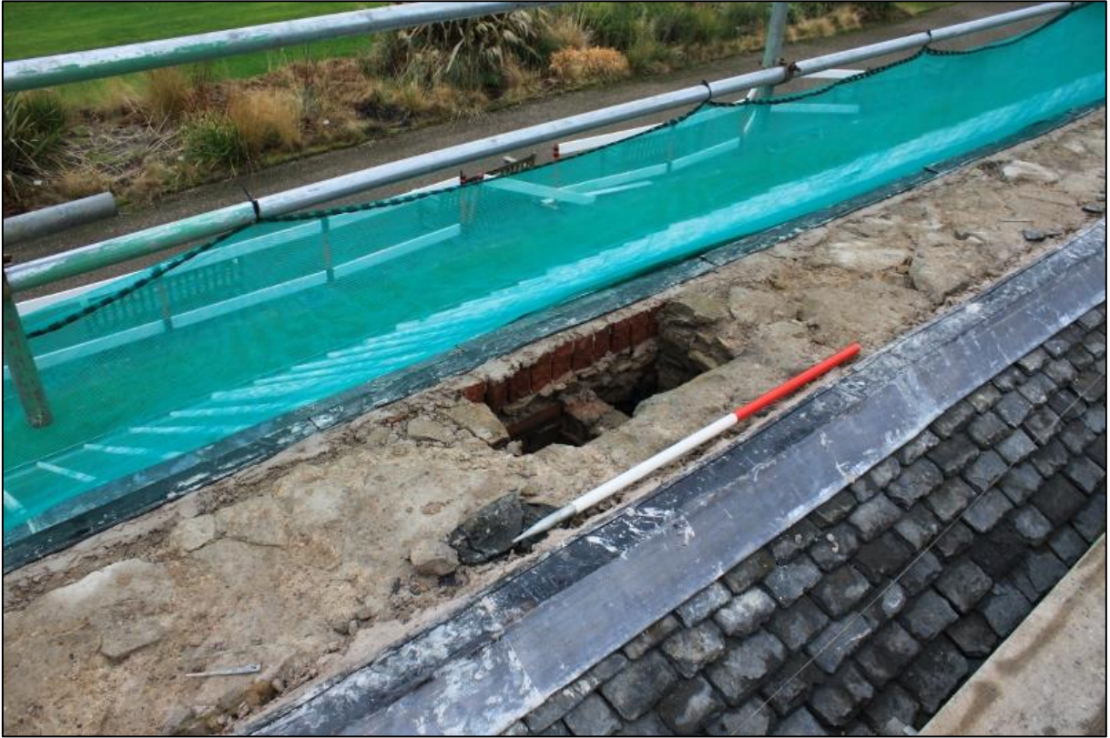
Figure 7a: Flues [027] and [028], partly dismantled at upper levels
