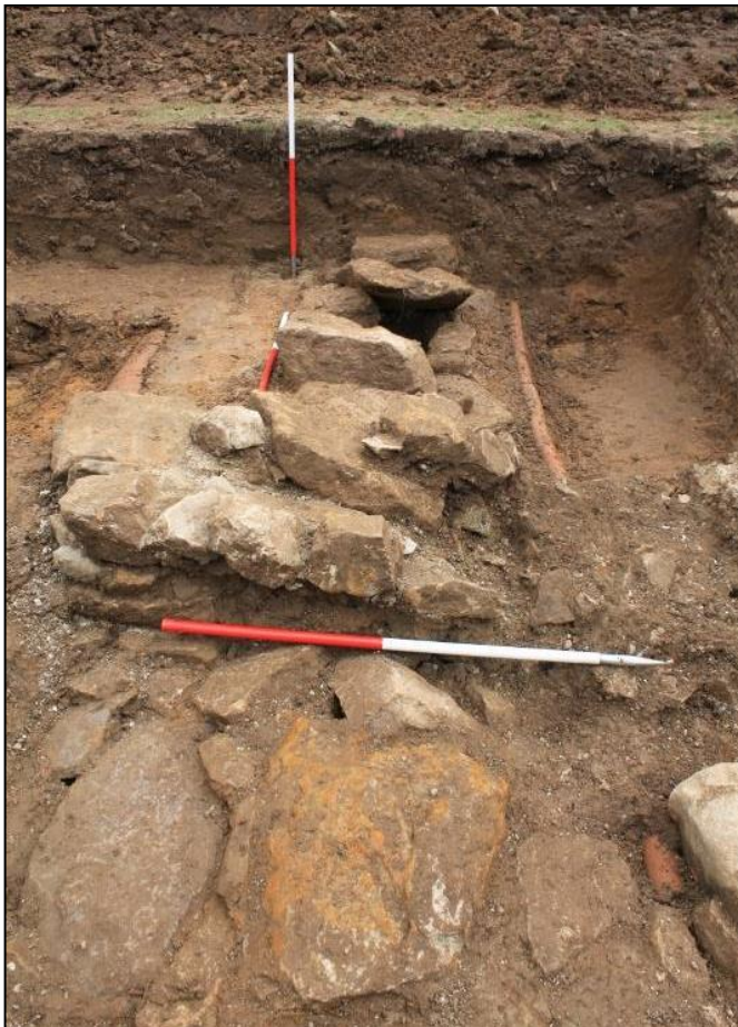
Figure 10b: Culvert [010] running through base of wall [008], taken from the southwest
