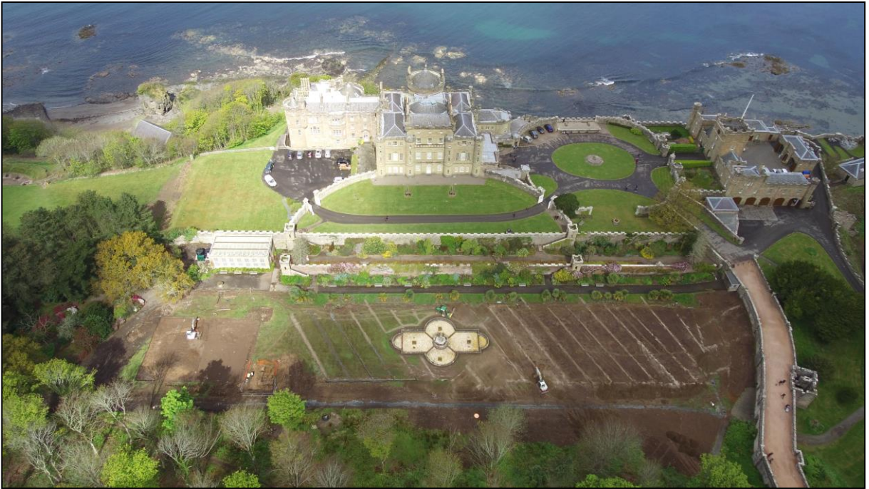
Figure 4a: Shot of Fountain Court from the southeast showing new drainage trenches, supplied by National Trust for Scotland
