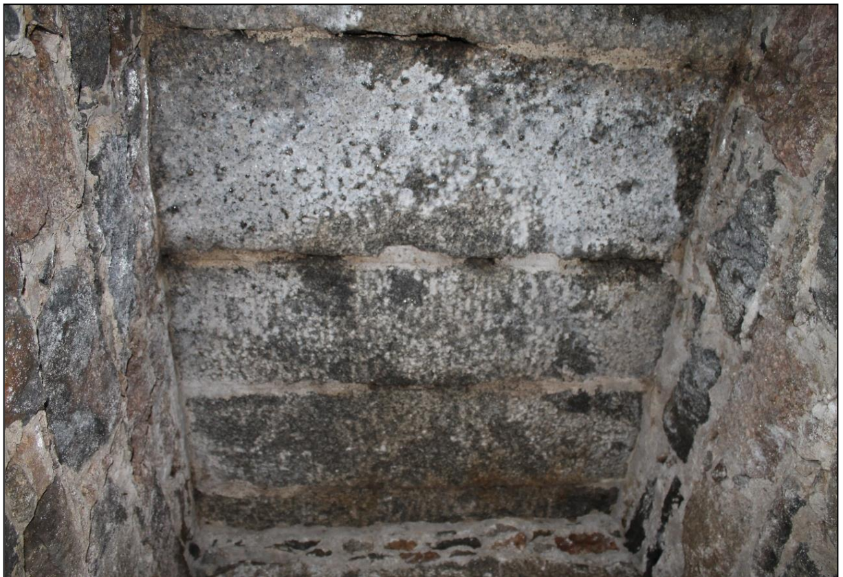
Figure 10b: Granite block entrance passageway ceiling
