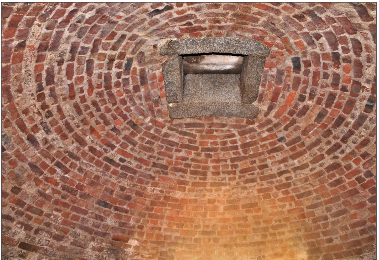
Figure 12b: Red brick dome roof with central square roof-light
