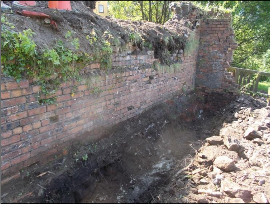
Figure 6a: Post excavation view of Trench 2. From the N.
