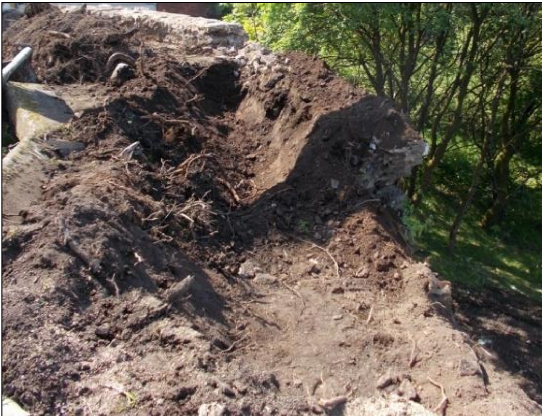
Figure 5b: Post excavation view of Trench 1 with Kerbstones in background. From the NNE.
