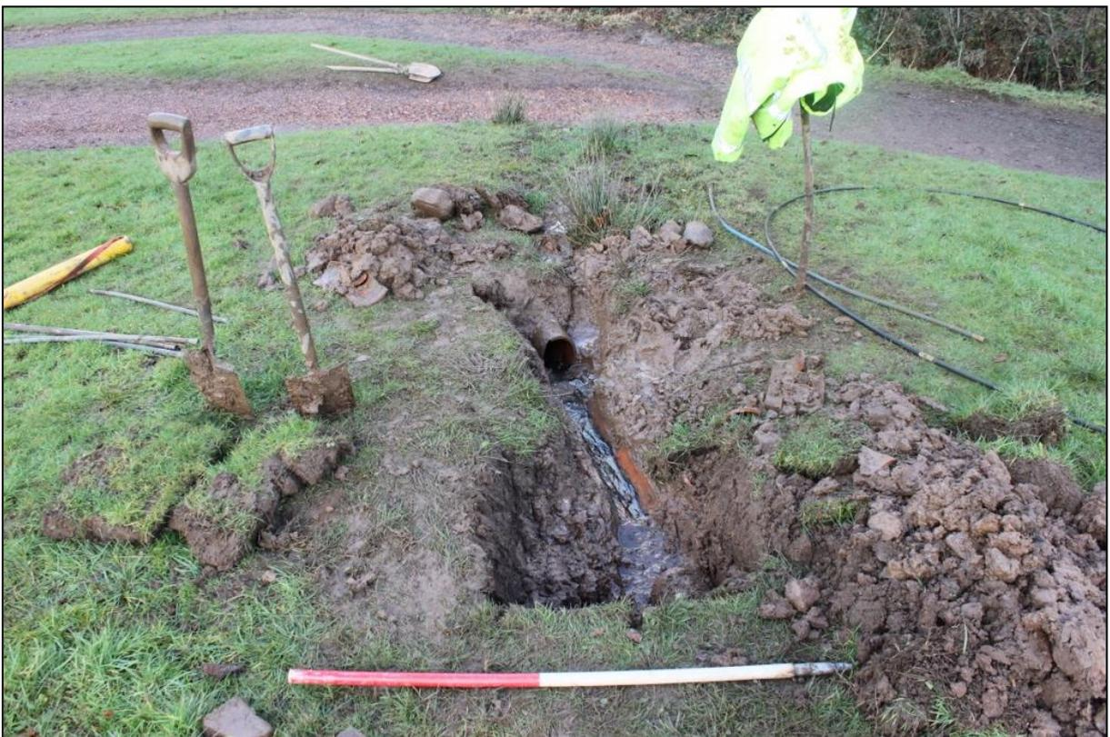
Figure 3: Damaged length of drain exposed during initial repair work (Area F).
