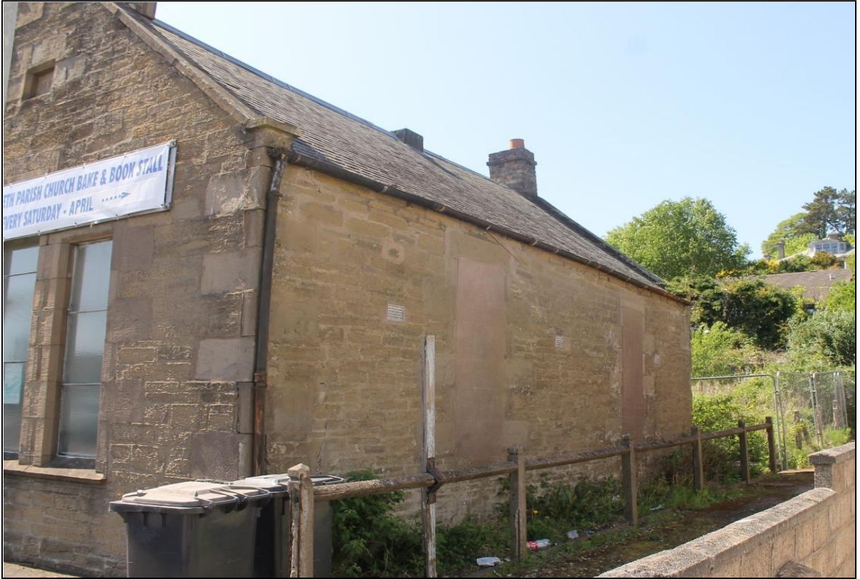
Figure 7a: Northeast elevation showing the two blocked windows
