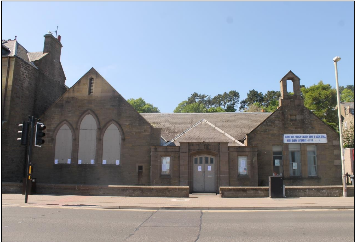
Figure 2a: Front southeast elevation
