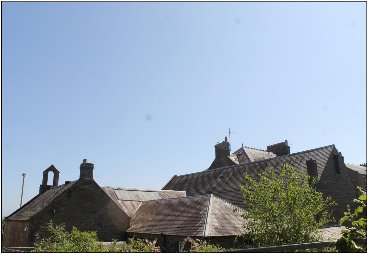
Figure 9a: Showing the red brick of the late-nineteenth century extension and the roofline
