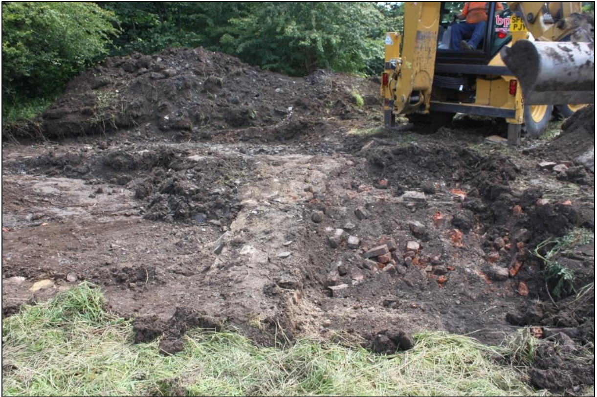
Figure 2a: Site being opened up by machine. Cottage walls and demolition layer (009) visible. From the NW.
