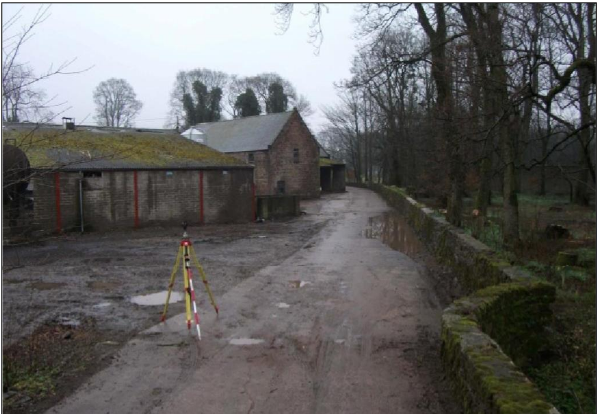
Figure 5b: Building A from the northeast
