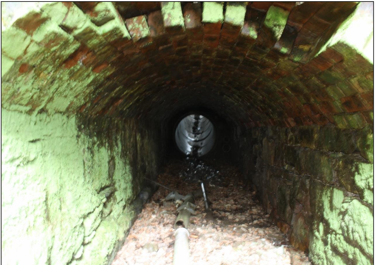
Figure 17a: The earlier, possibly 19 th century tunnel for the lade.
