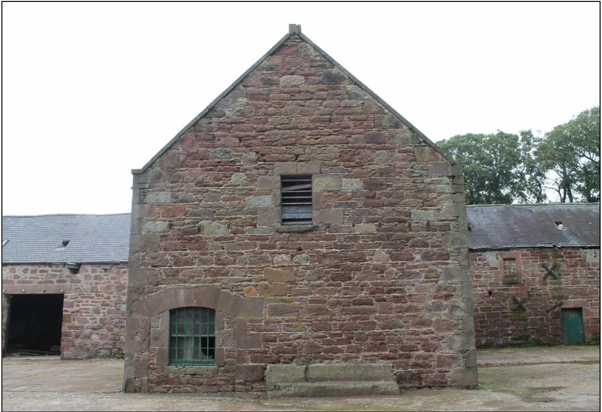
Figure 12a: Southwest elevation of the South Barn.
