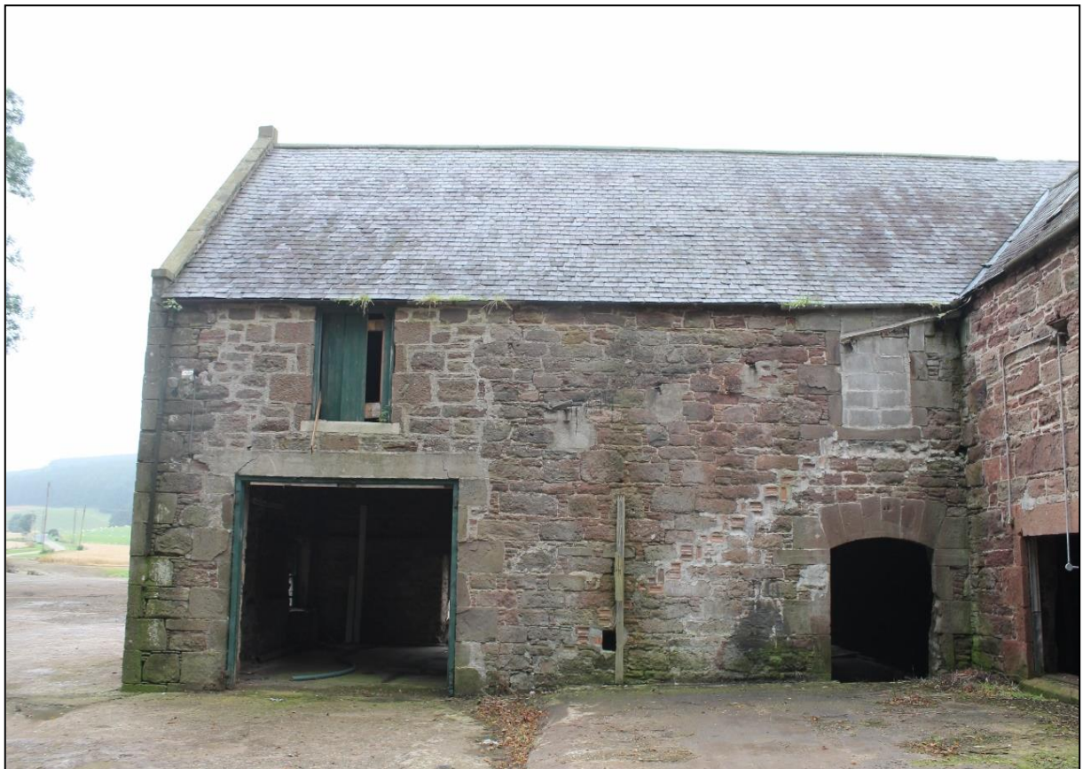
Figure 12b: Southeast elevation of the South Barn.
