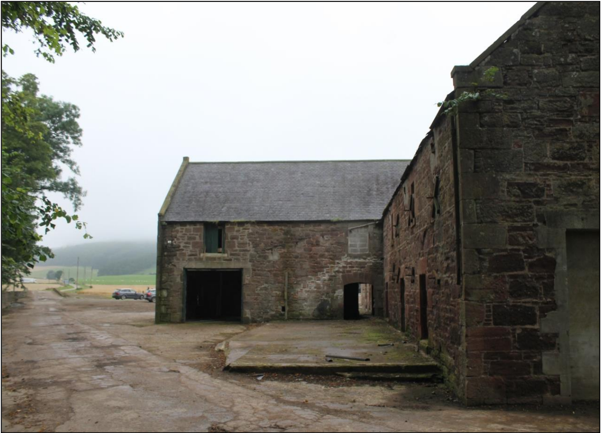
Figure 9a: Structure removed from the southwest side of the South Barn
