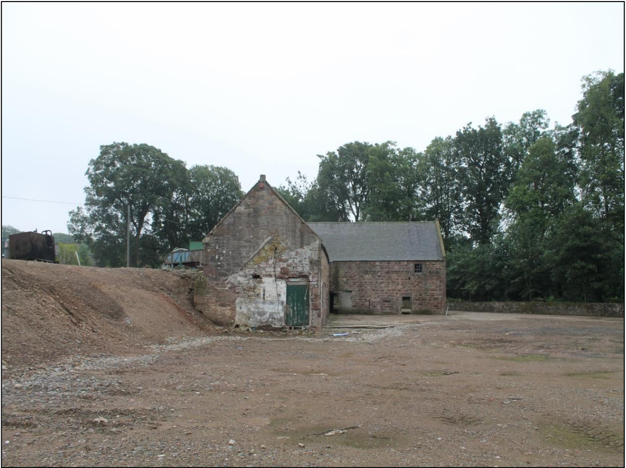
Figure 8a: Area where Building A would have stood. Evidence on the northwest elevation of the North Barn demonstrates where the two buildings adjoined.
