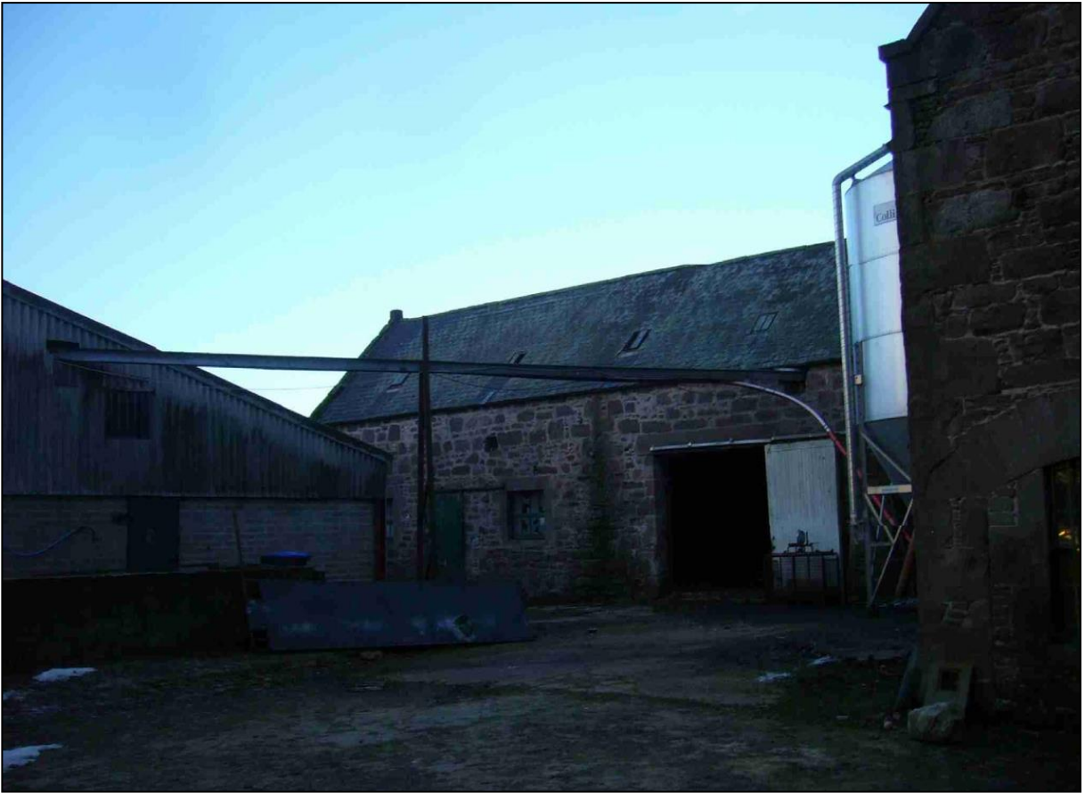
Figure 4a: Building A, adjoining to the North Barn.
