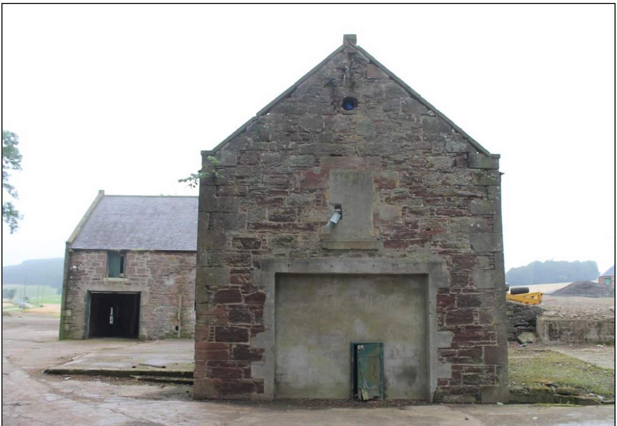
Figure 13b: Southeast elevation of the South Barn.
