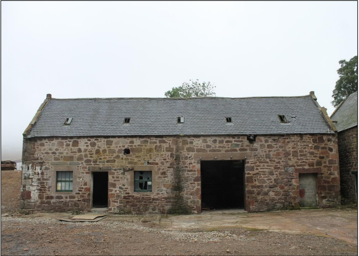
Figure 10a: Southwest elevation of the North Barn
