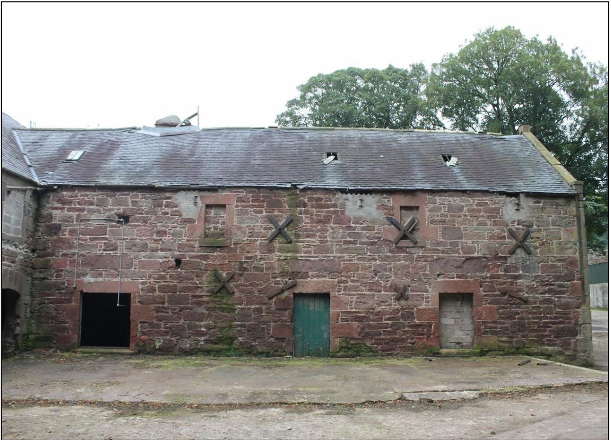
Figure 13a: Southwest elevation of the South Barn.
