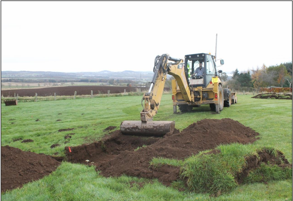
Figure 4a: A CAT 432E was used to excavate the trenches
