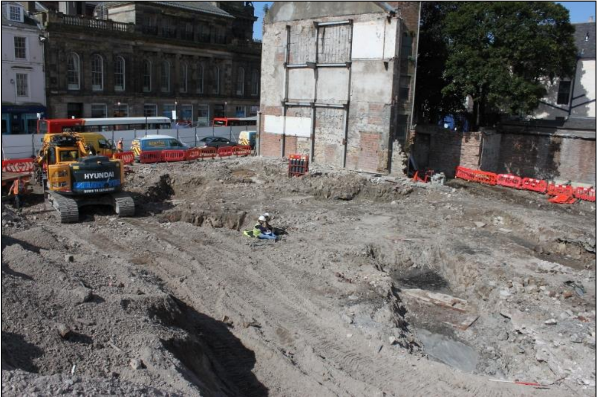
Figure 3a: General shot showing made ground (001) from the east
