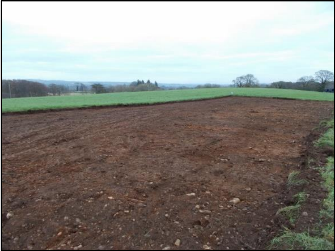
Figure 7: Post excavation view of development area. Taken from the W.
