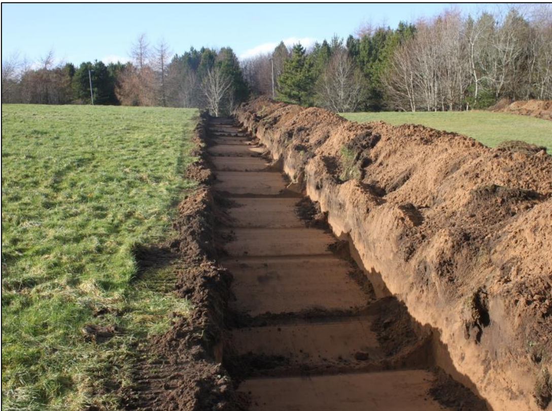
Figure 6b: Post excavation view of T9 from the E
