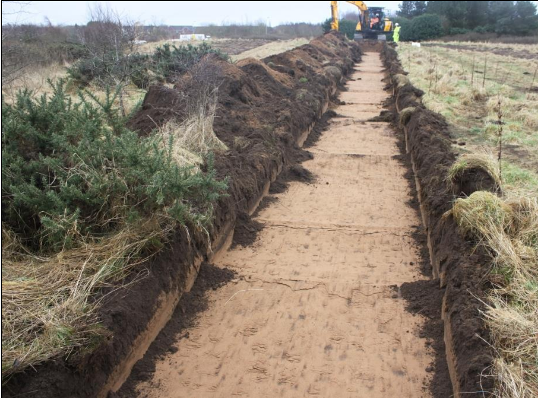
Figure 7a: Post excavation view of T26 from the NNE
