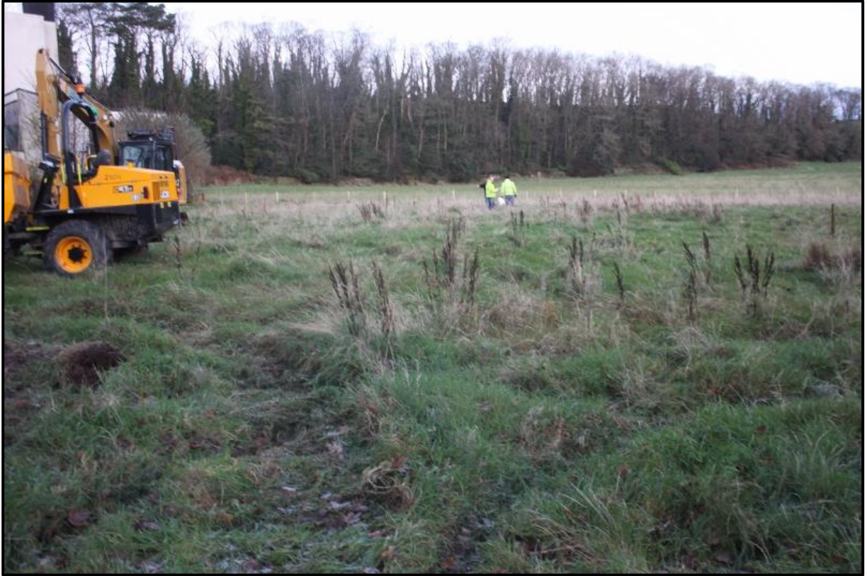
Figure 3a: Pre excavation view of development area. From the southeast
