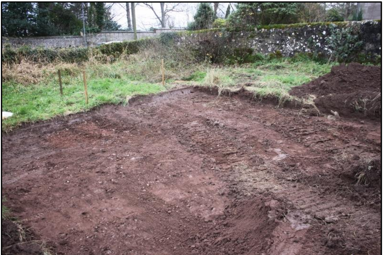
Figure 3b: Post excavation shot of south end of footprint showing subsoil (005). Taken from the northwest.
