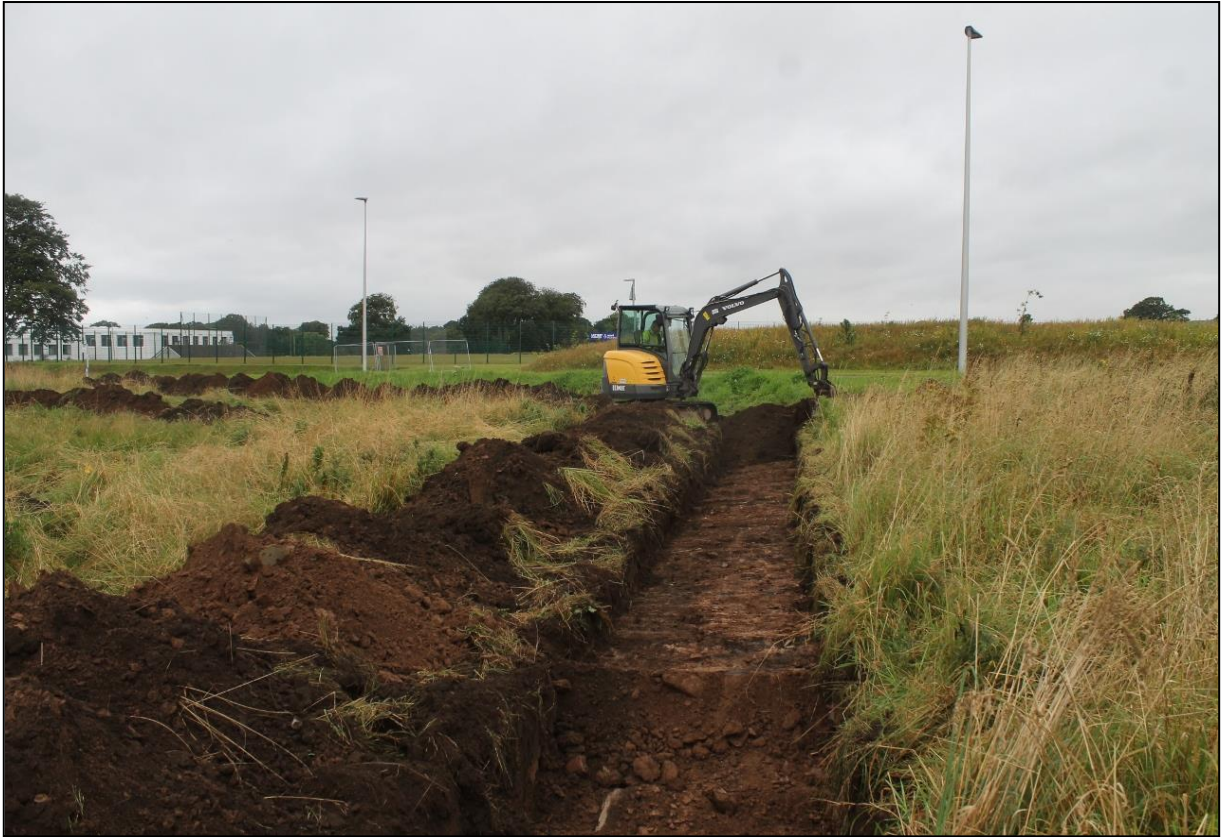
Figure 3a: Excavator used was a Volvo ECR48C.
