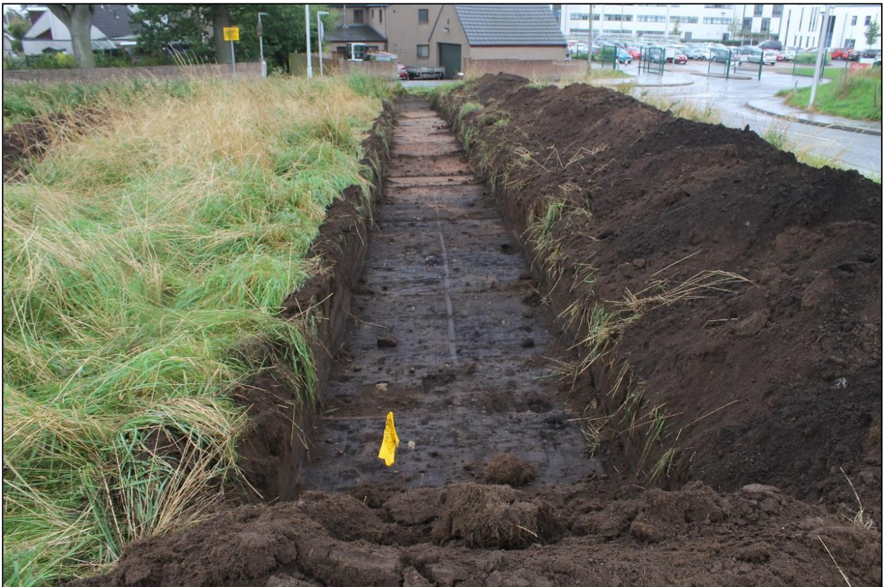
Figure 4b: Trench 7 demonstrating context (003), possibly representing early peat formation.
