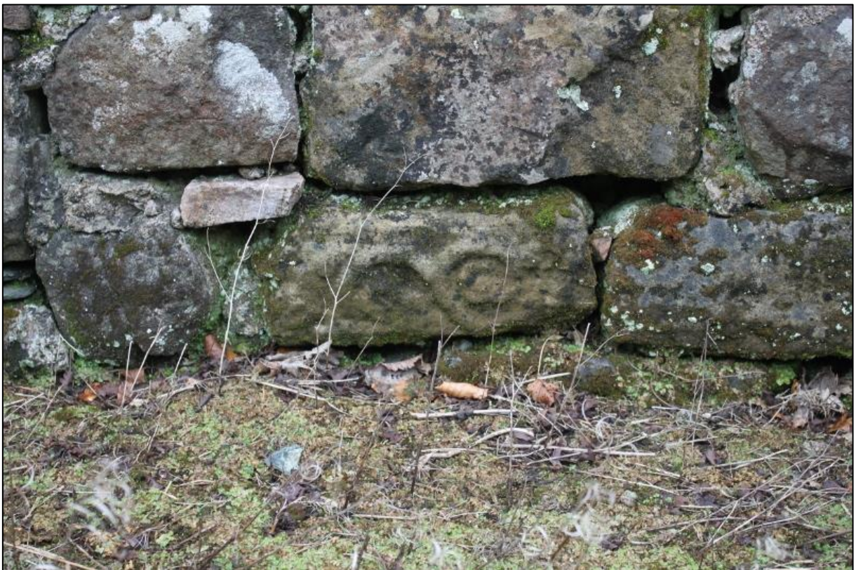
Figure 4b: Interior, South Elevation: Re-used carved stone (?fragmentary cross-slab) within Fabric 6 blocked doorway
