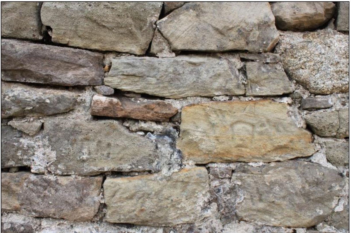
Figure 8b: Fabric 6, Carved stones incorporated into blocked doorway in South Elevation
