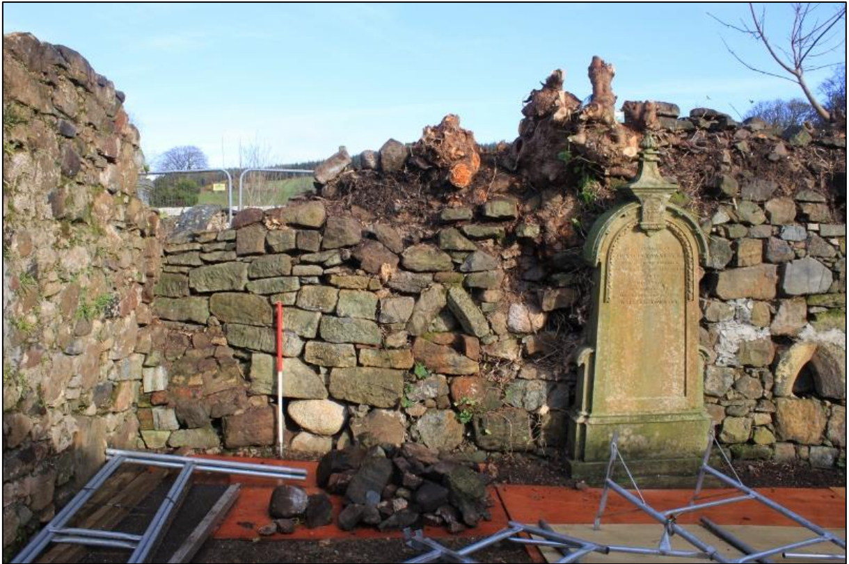
Figure 2a: North-west corner (internal elevation) prior to works commencing, with squared rubble repair pushed out of alignment and root masses clearly visible at wallhead
