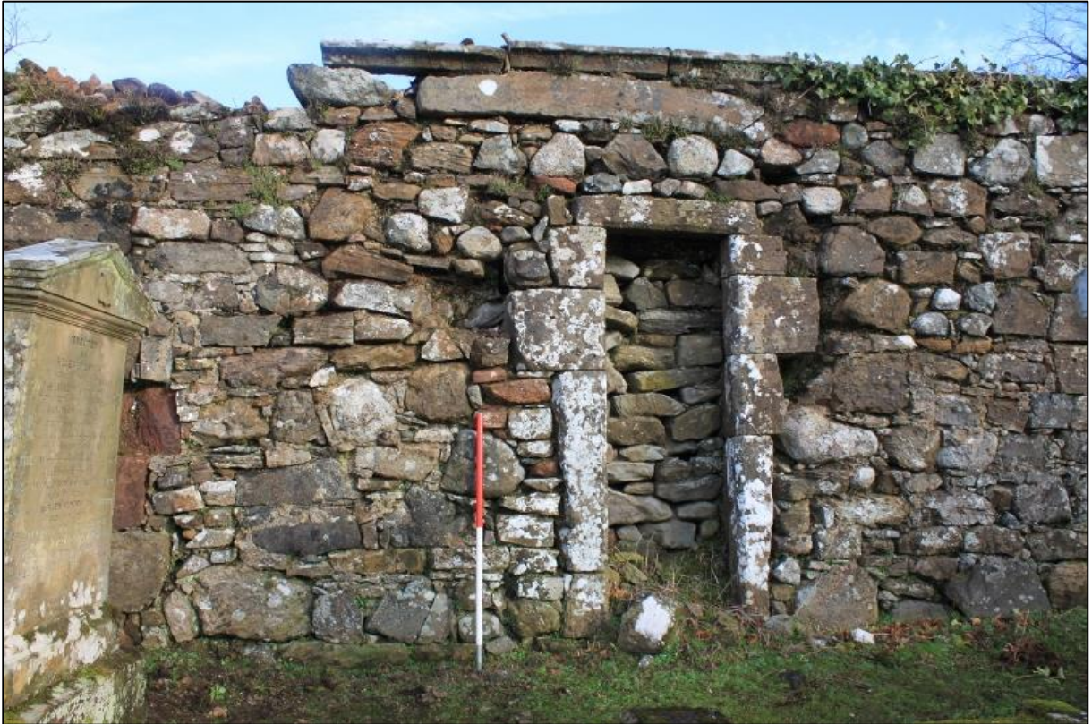
Figure 8a: Fabric 6, Blocked opening (?doorway) in South Elevation
