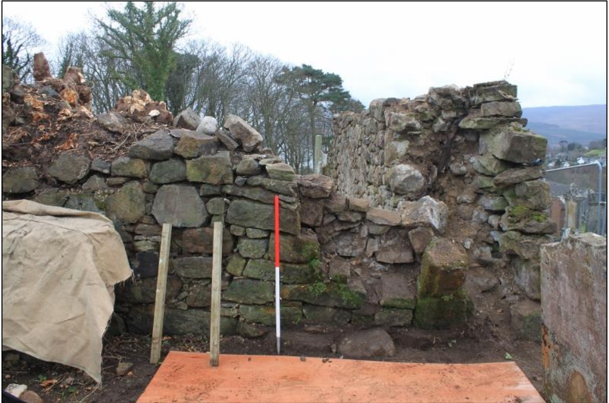
Figure 3a: North-west corner (external elevation): rubble cleared, threshold stone (broken) revealed in basal course with in situ rybat to west (two displaced rybats above)
