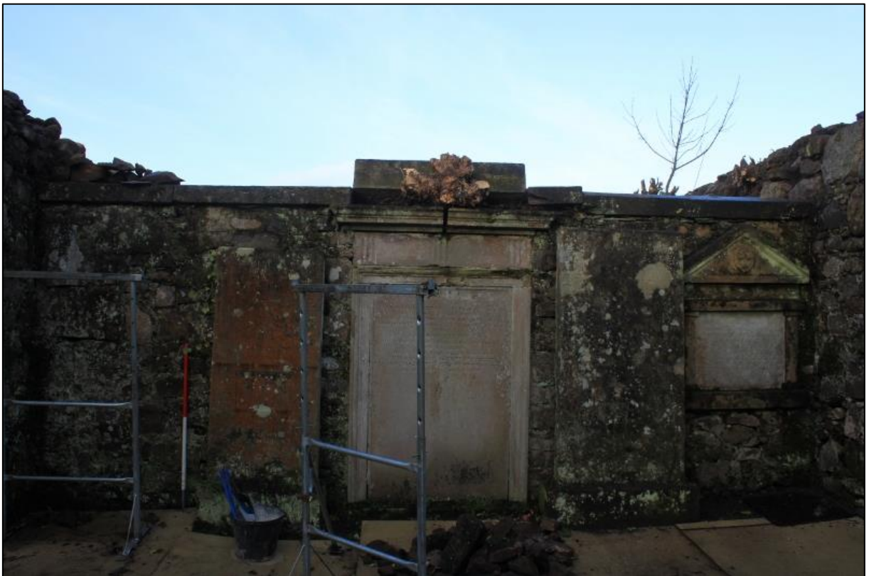
Figure 7b: Fabric 5, East Elevation of North-South Cross-Wall
