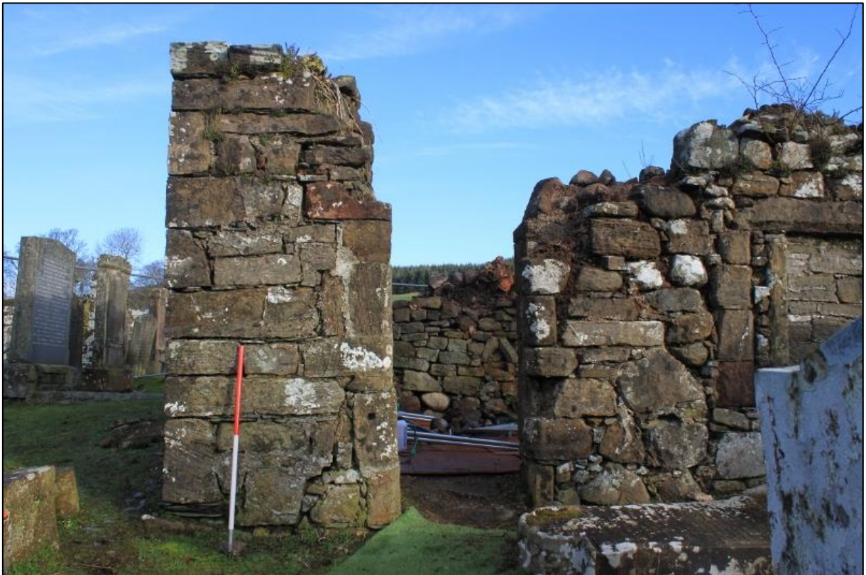
Figure 6b: South Elevation, W end: Fabric 3 in doorway
