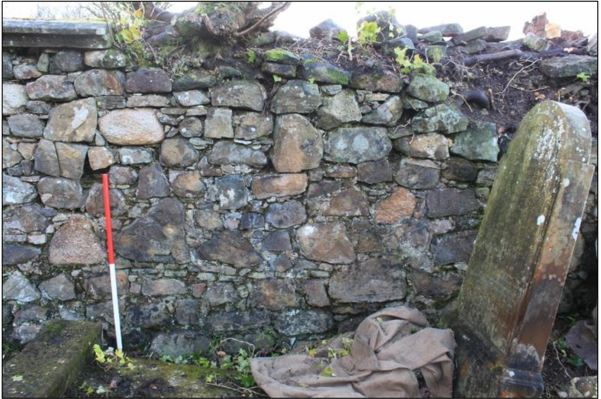
Figure 5a: North Elevation (external elevation, approx. 5-6m east of west end): Fabric 1 in lowermost six courses, showing thin line of snecking stones overlying irregular, unworked blocks
