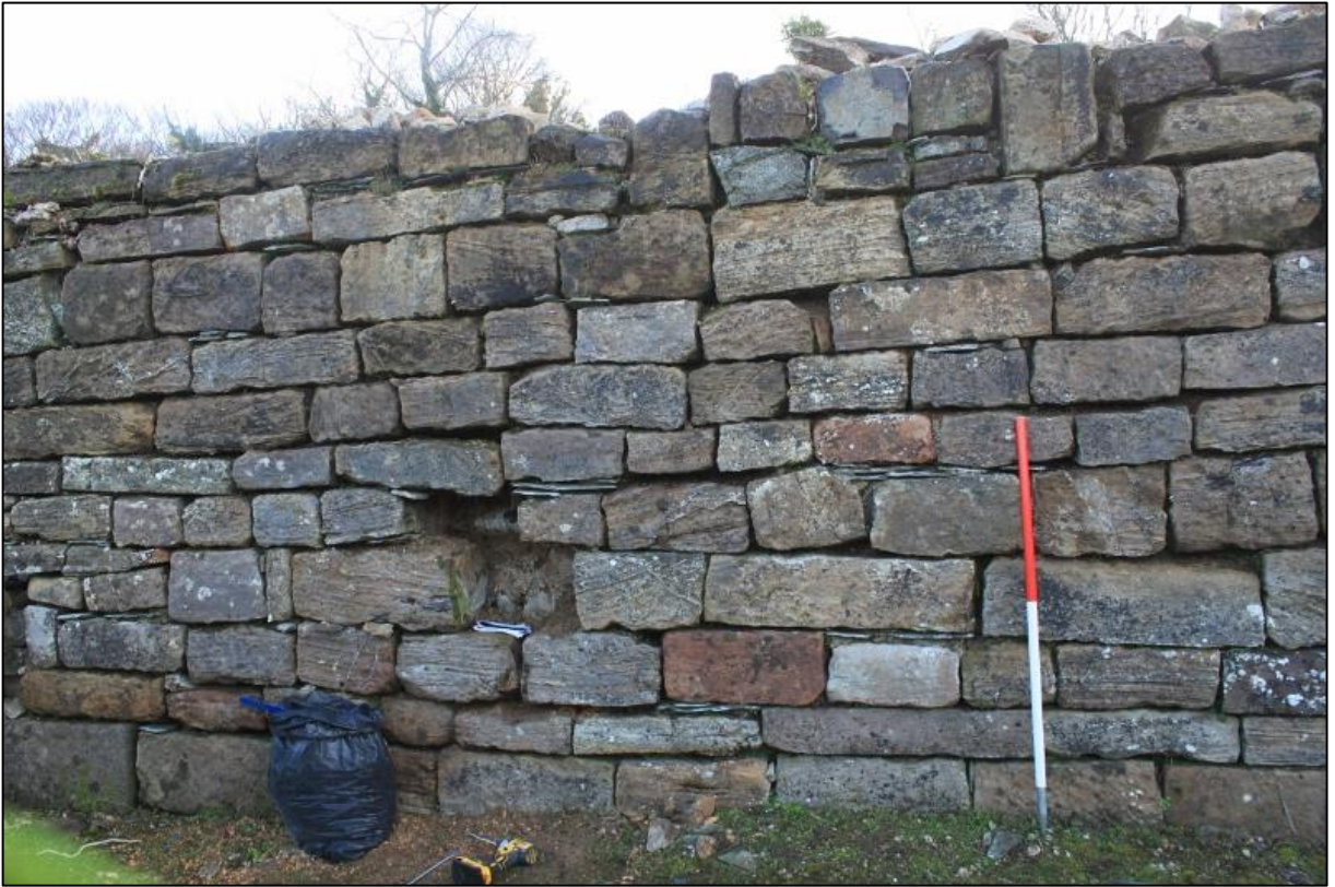
Figure 6a: West Elevation: masonry in Fabric 3, with slate pinnings clearly visible
