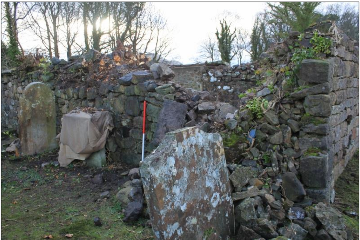
Figure 2a: North-west corner (internal elevation) prior to works commencing, with squared rubble repair pushed out of alignment and root masses clearly visible at wallhead
