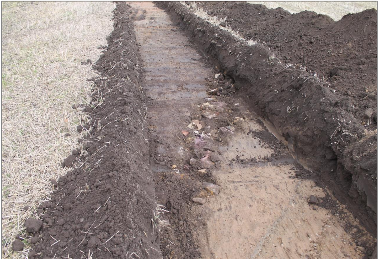
Figure 9a: Showing rubble field drain (010)
