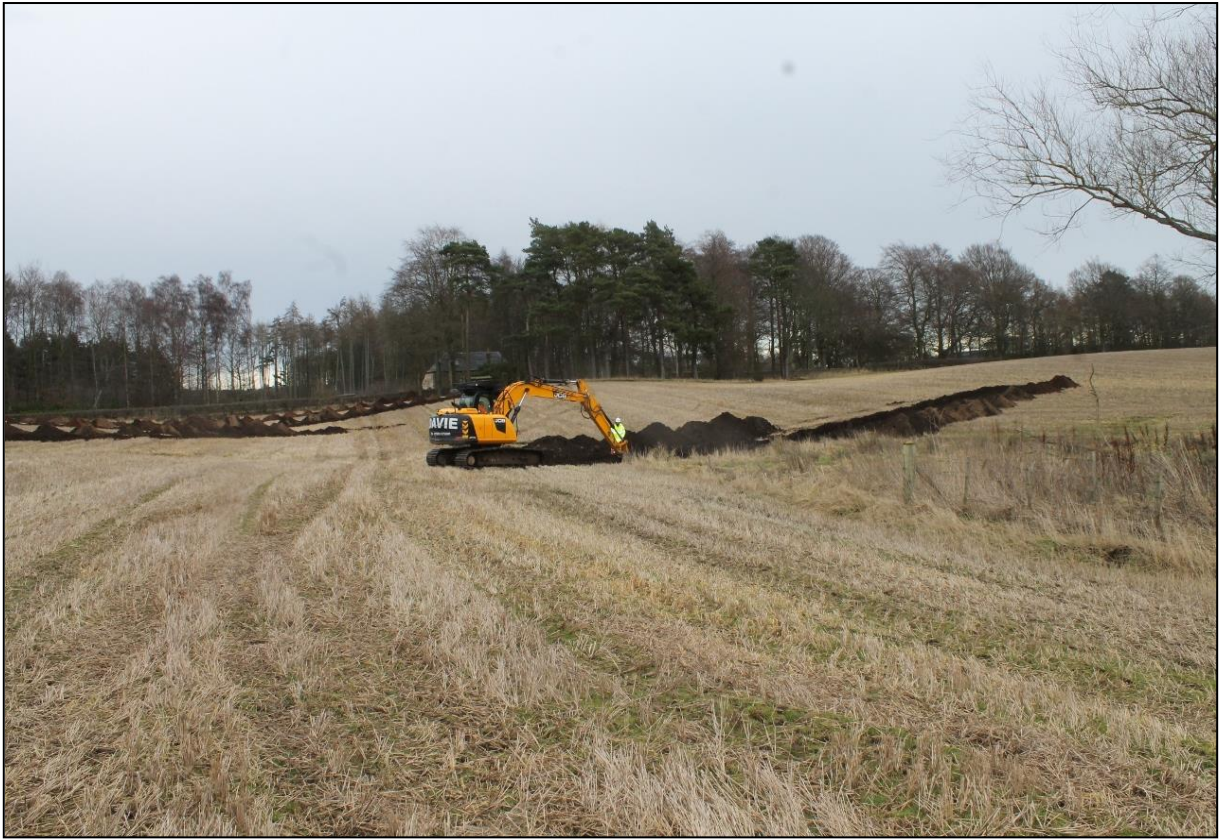
Figure 3a: Working shot showing JCB JS145 excavator.
