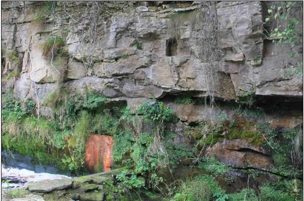
Figure 4b: View of Putlog Hole close to the ENE end of Basin 2. From the SSE.
