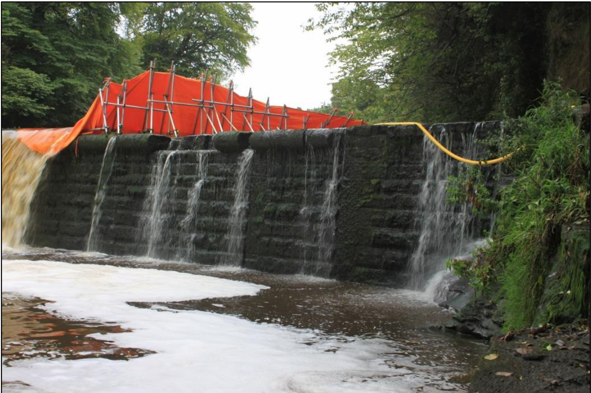
Figure 6b: Close up view of the Weir structure from the NE.
