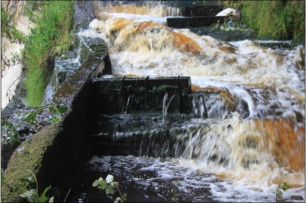
Figure 4a: Close up view of Riser A. From the ENE.
