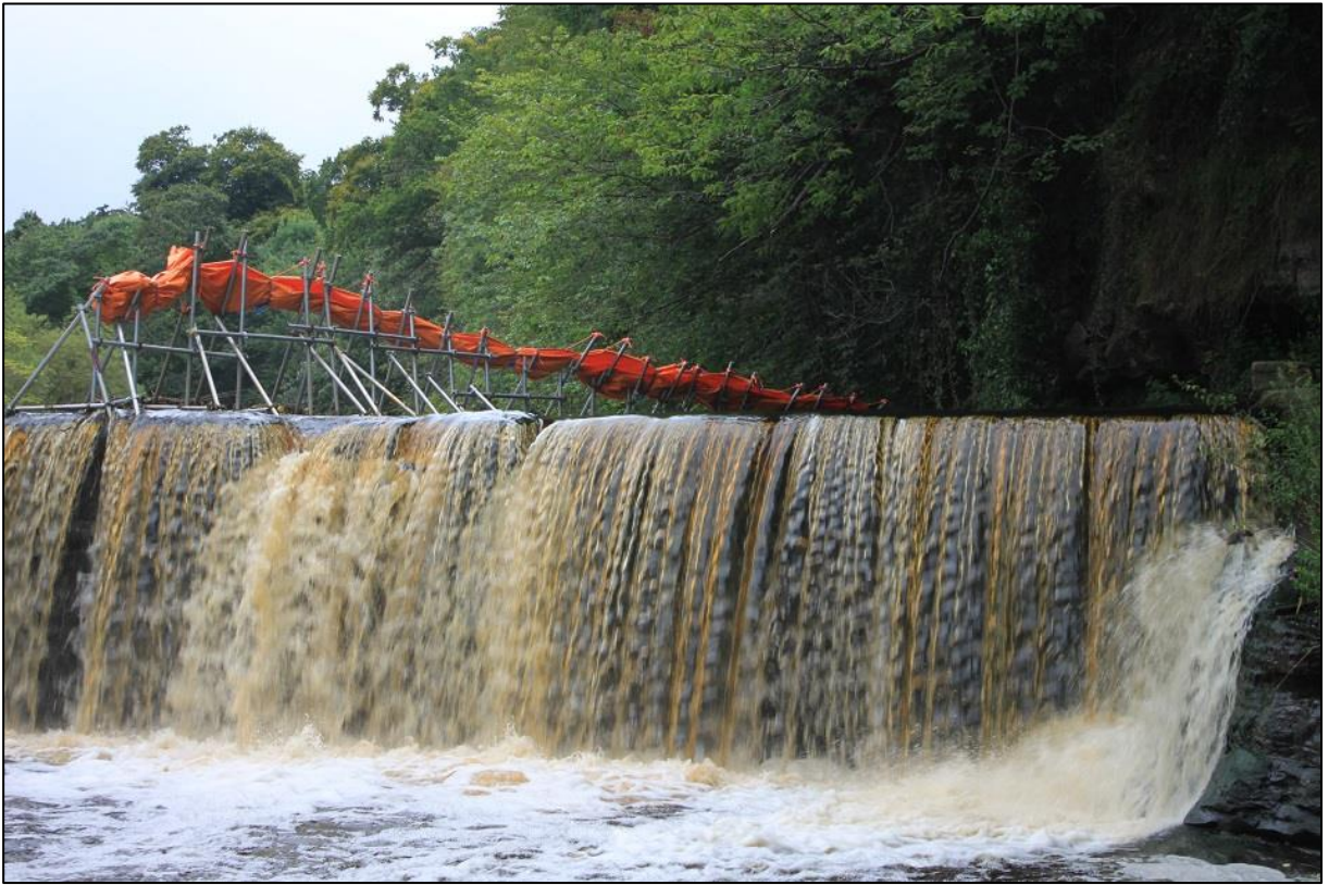
Figure 2a: View of the Weir before works commence. From the W.
