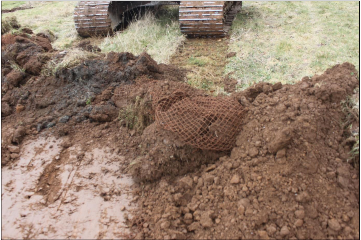
Figure 3a: Orange netting (006) under topsoil, seen along length of excavation.
