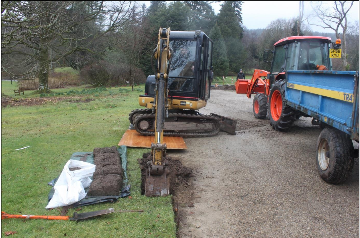
Figure 2b: Pit 5 (E) Machine excavation narrow toothed bucket. From SE
