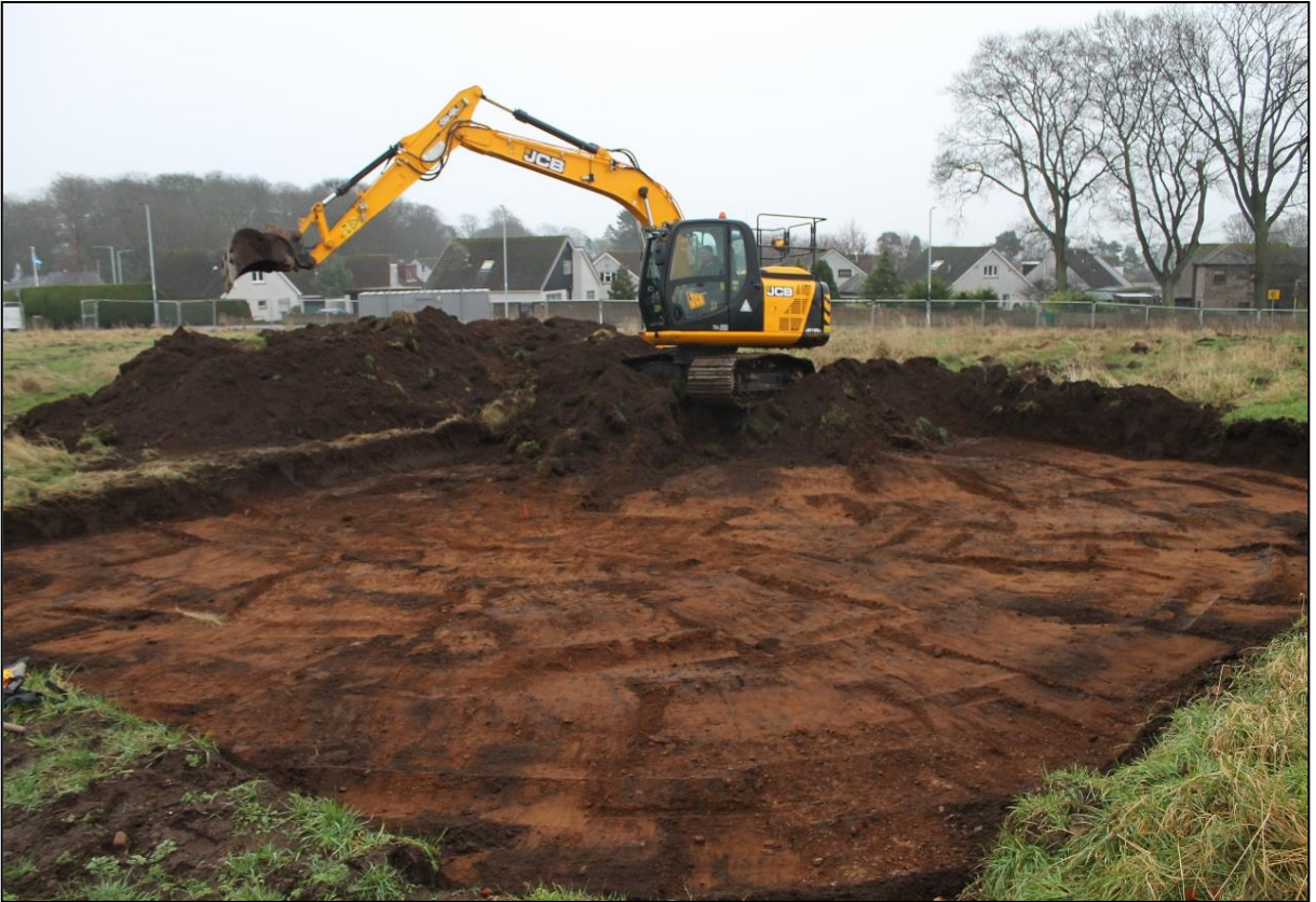
Figure 4a: Excavator used was a JCB JS130.
