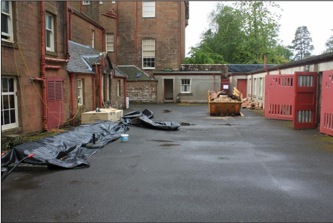
Figure 4a: Pre excavation view of the Courtyard and Bobby's Building. From the NE.
