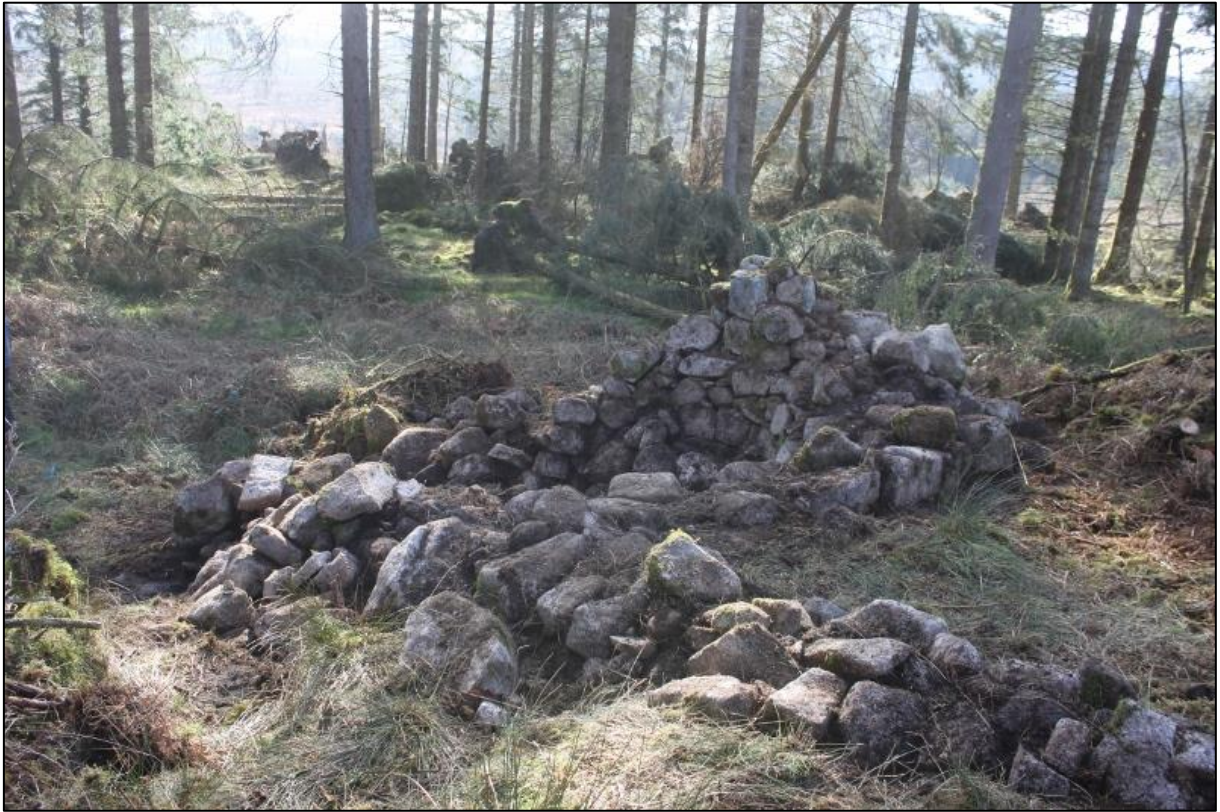
Figure 5a: Shot showing difference in height between barn [001b] on the right and kiln [001a] on the left, set into natural slope
