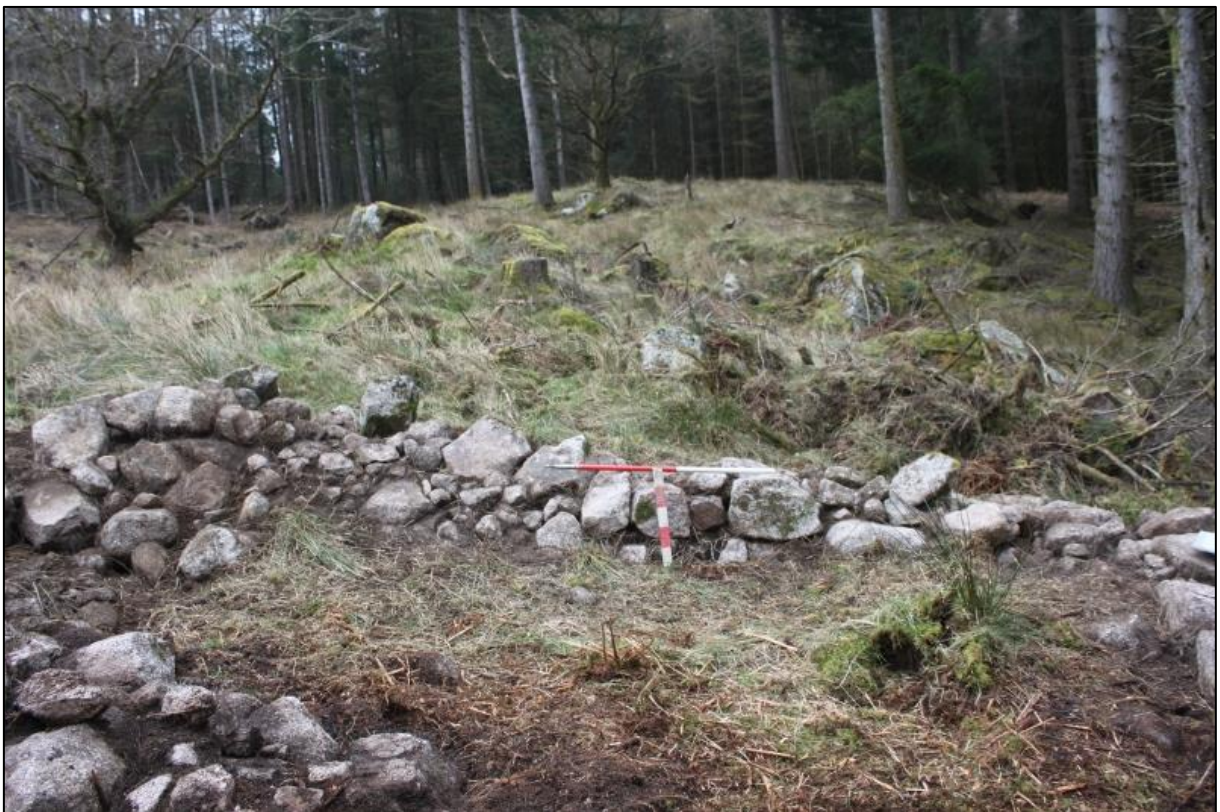
Figure 4b: Detail of eastern wall of barn [001b] from the west-northwest
