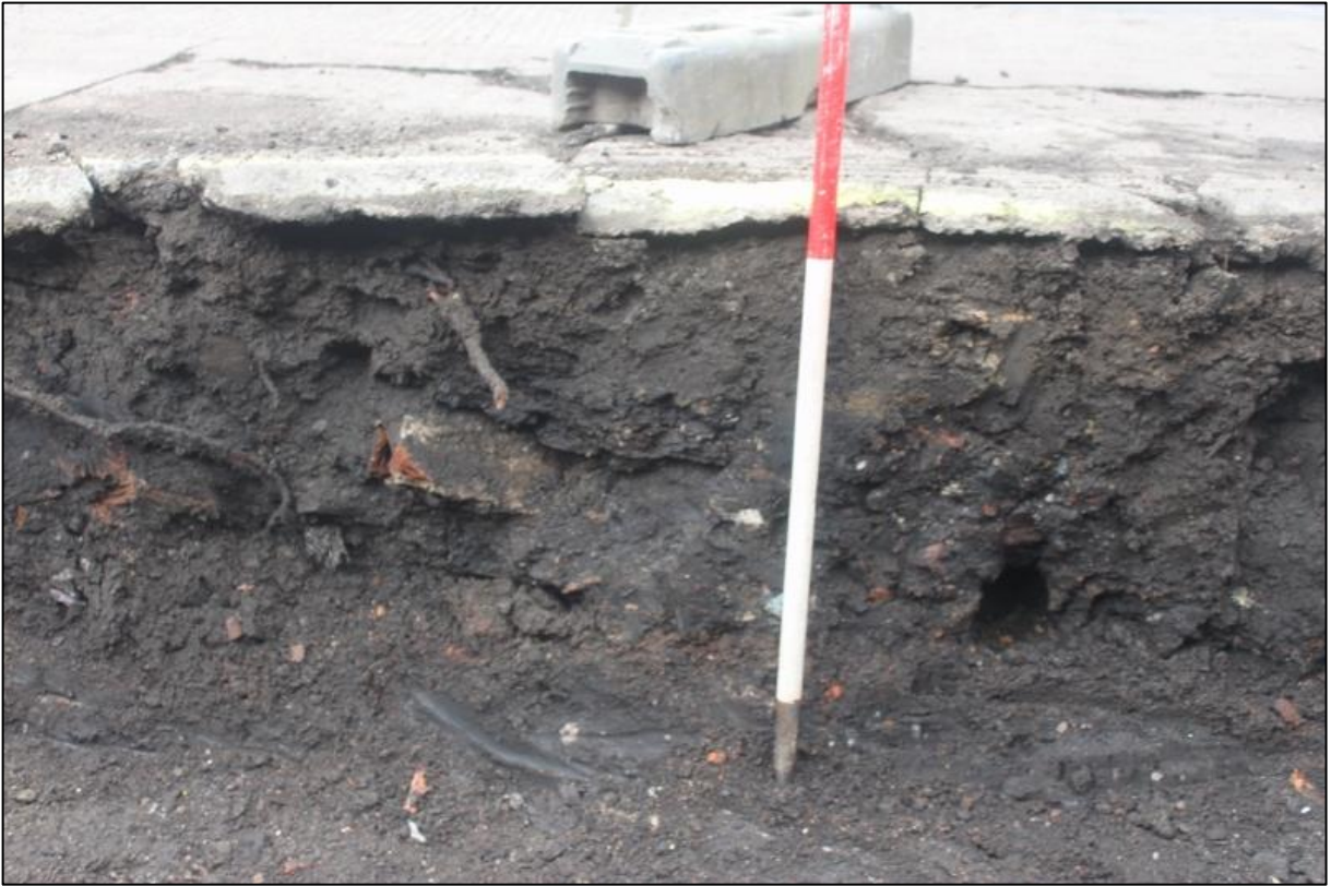
Figure 4a: Section shot of foundation trench adjacent to pavement. Photo taken from the southeast.
