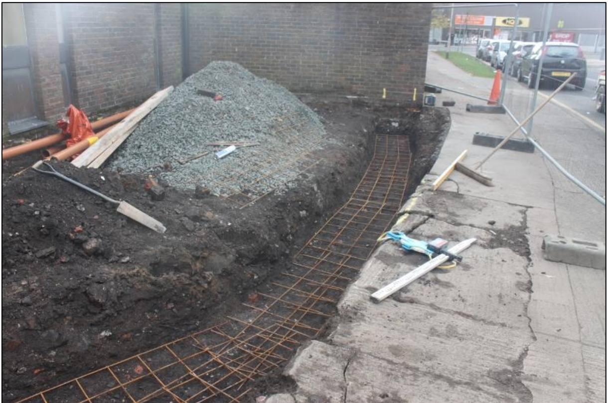
Figure 3b: Post-excitation shot of foundation trench. Photo taken from the north.
