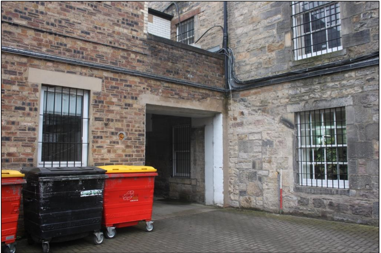
Figure 17a: View of raised corridor linking Building 3 to 24 Forth Street. From the NW.
