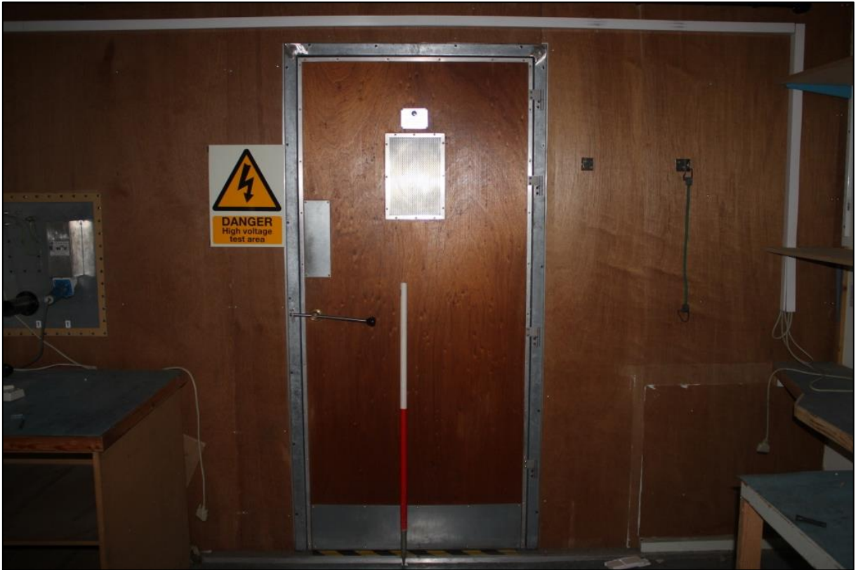
Figure 16a: View of S facing wall within Room 17, Building 3. From the S.
