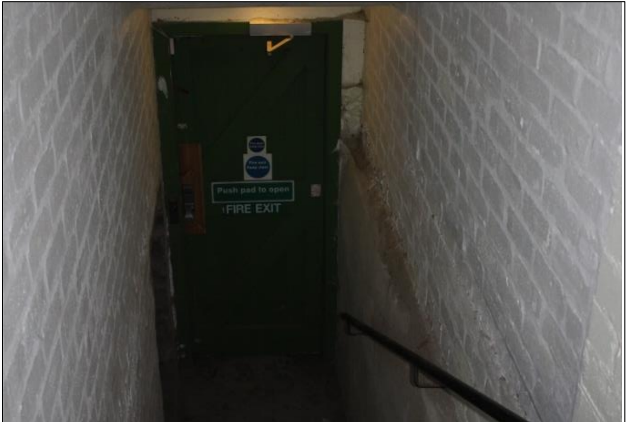
Figure 15a: Emergency stairs/door within basement level of Building 3. From the S.
