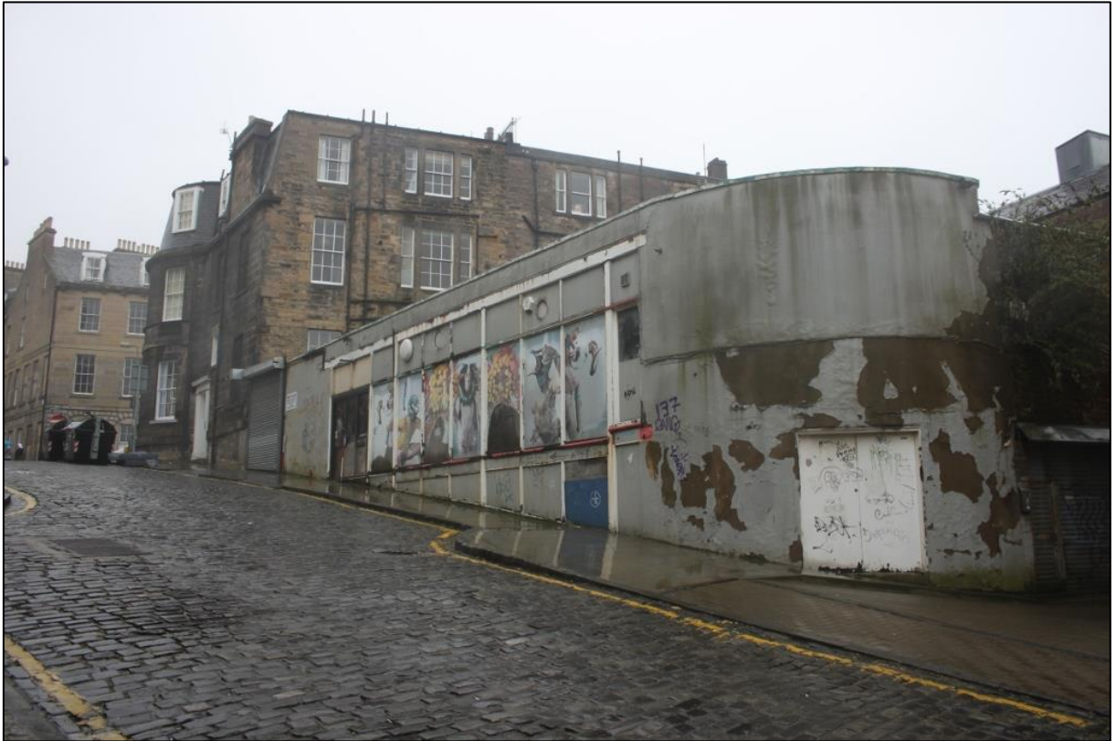
Figure 9a: General view of 14-16 Union Street. From the SSW.
