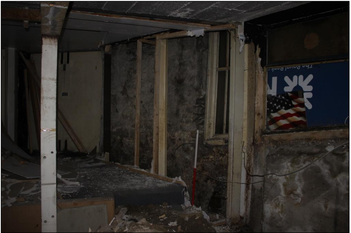
Figure 11a: Room of 10a within Building 1. From the SSW.
