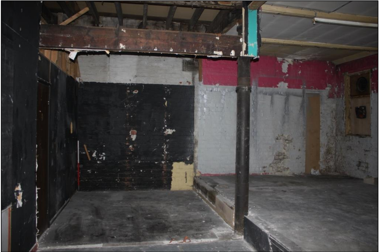
Figure 10a: View of Room 4 within Building 4. From the E.
