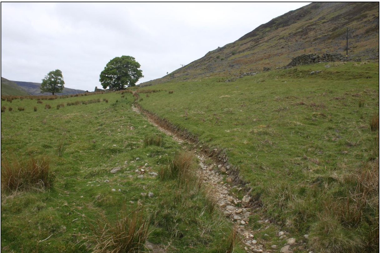
Figure 5b: Ditch [004] after reinstatement complete from the east.
