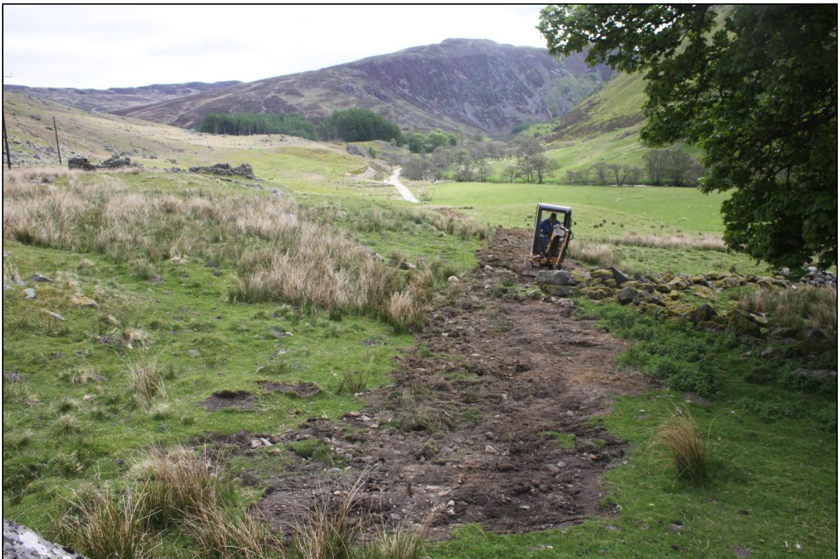
Figure 4b: Ditch [003] after reinstatement complete from the west
