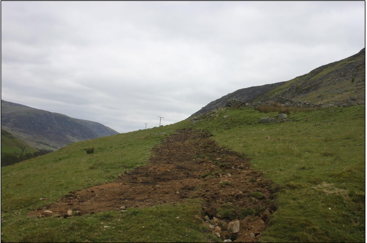
Figure 5a: Pre-Reinstatement of ditch [004] from the west.
