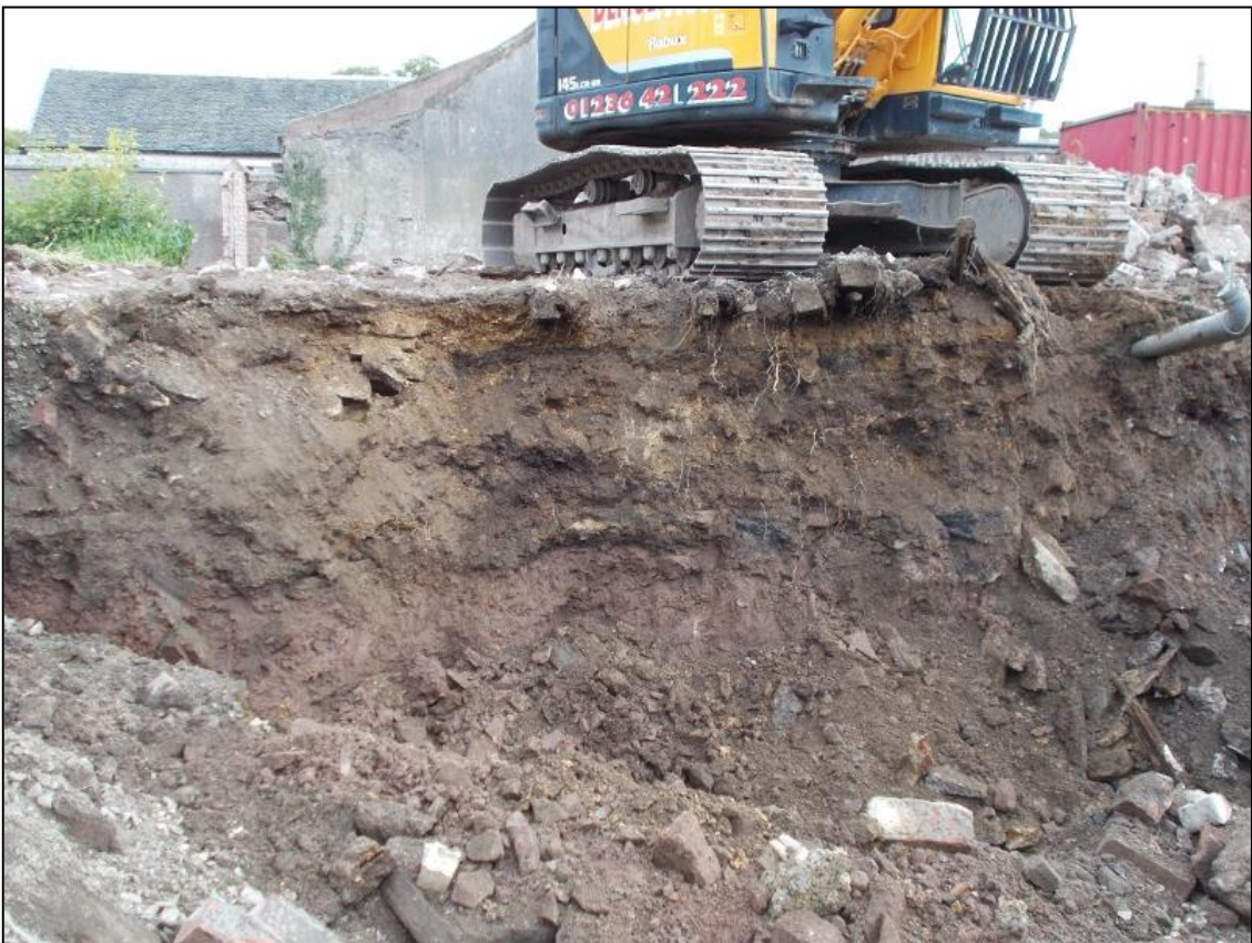
Figure 3b: South facing section along rear yard, after north wall of SW building removed
