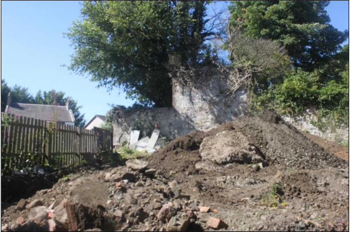
Figure 5a: General shot of site taken from the south.
