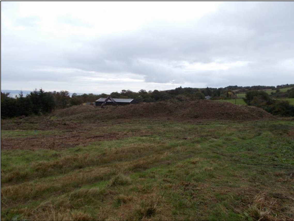
Figure 5a: Shot towards bund around substation from the west
