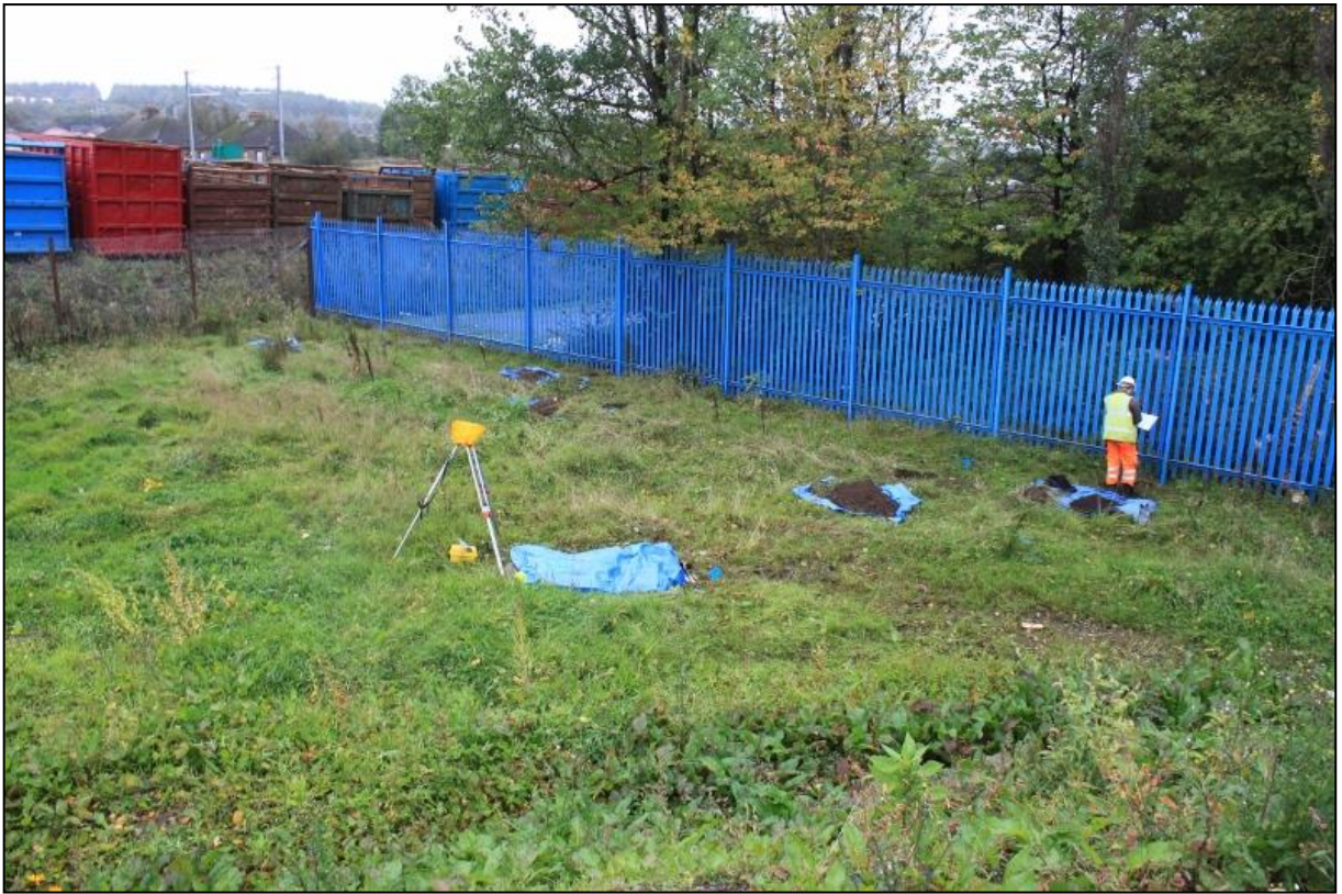
Figure 4a: TP array from N and palisade fence
