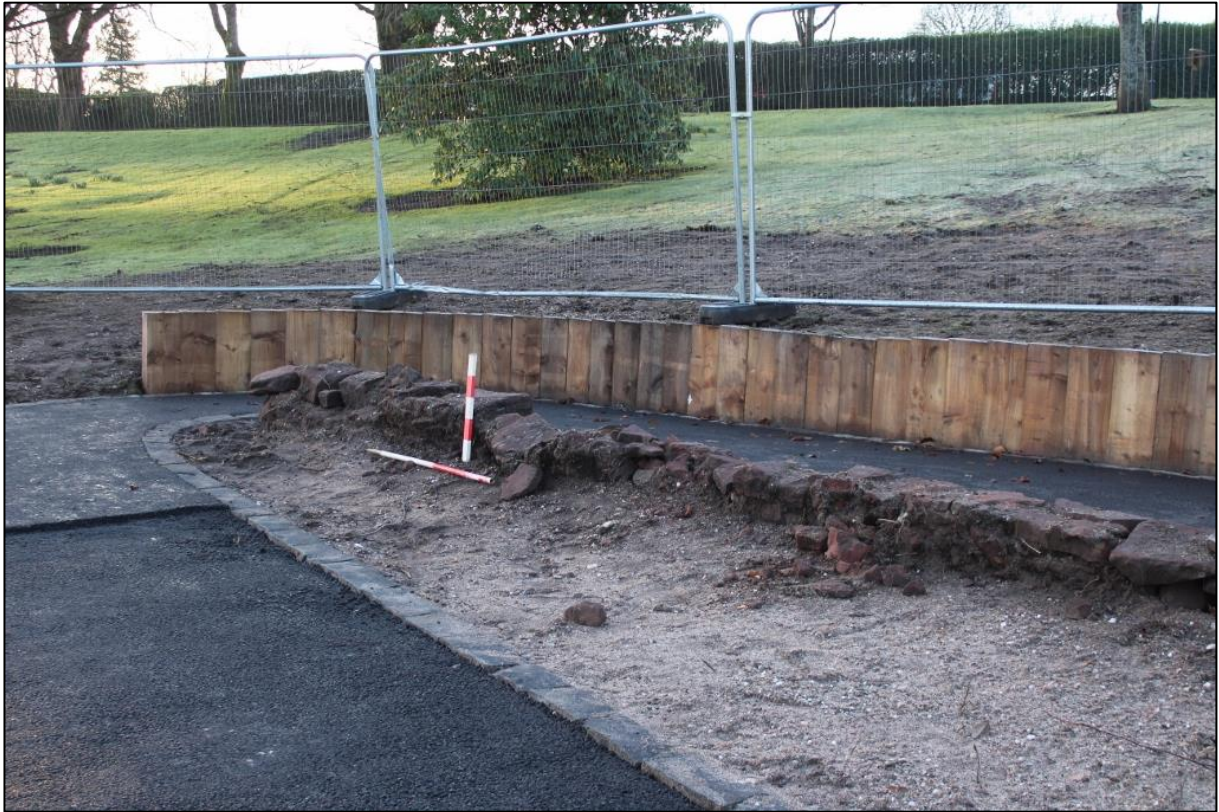
Figure 6a: View of the extension of wall [004] from the N.
