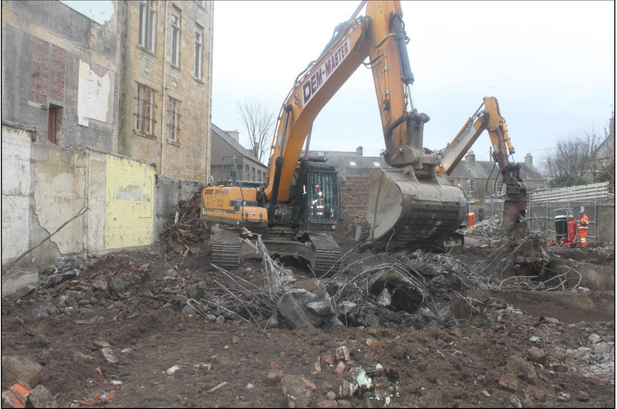
Figure 5a: Removal of foundation to the south of the development area.
