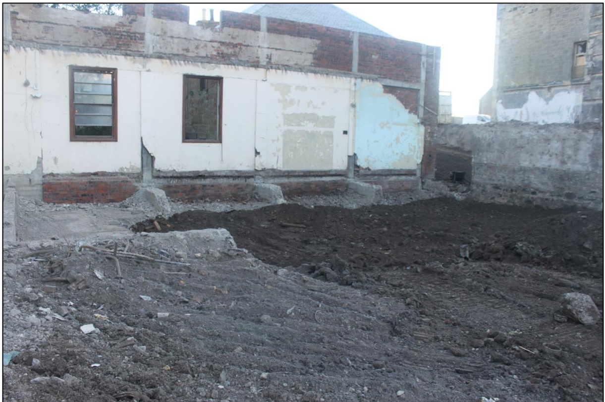
Figure 4b: Removal of foundation to the north of the development area.
