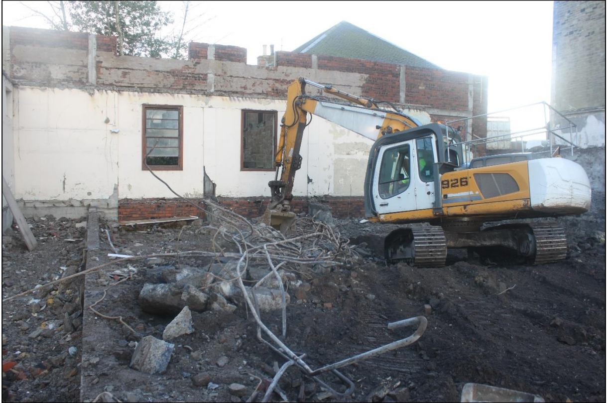
Figure 4a: Northern area post excavation.
