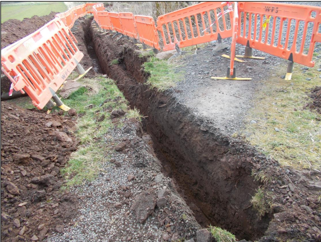
Figure 3b: Mid-excavation of trench cut through path (004) from northwest
