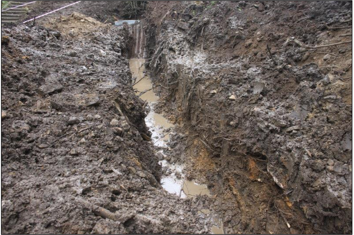
Figure 3a: Post-excitation shot of Drain 2 from the west.
