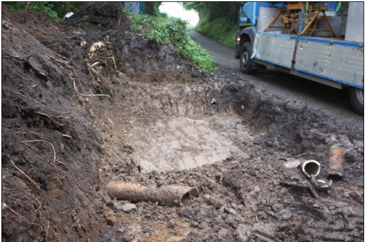
Figure 2b: General shot of Tank 1 from the east.
