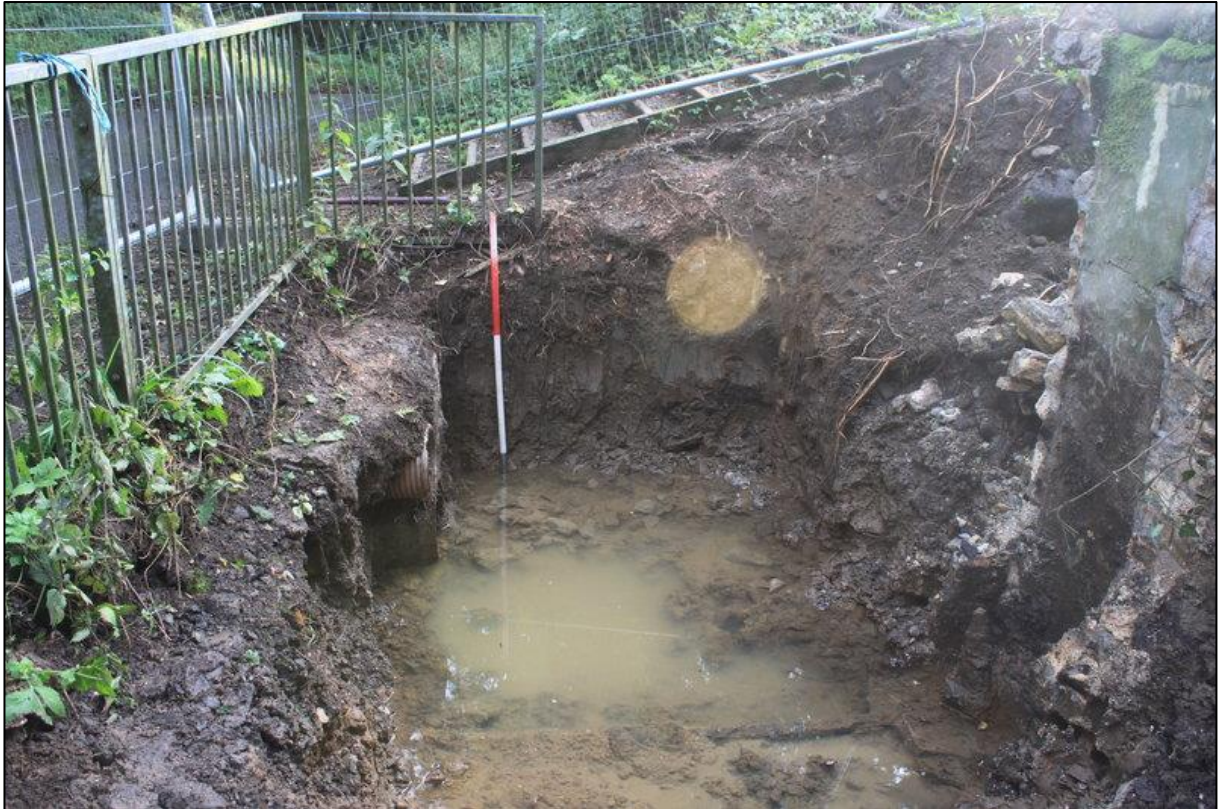
Figure 2a: Post-excitation shot of Manhole 1 from the west.
