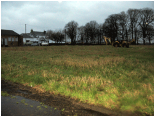
Fig. 3a: General Shot Pre-Ex of Site
