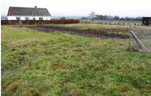
Fig. 3g: Backfilled trenches
