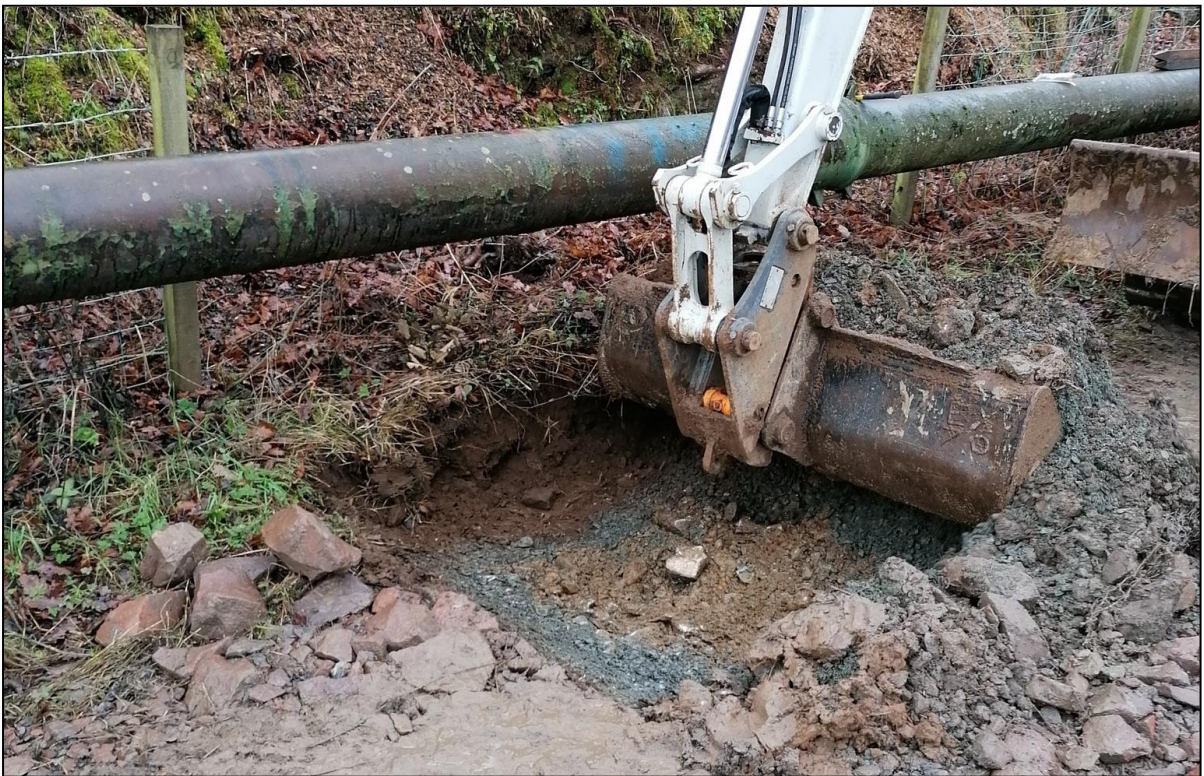
Figure 3b: Working shot of Pier 20 showing excavation through the access road. From E.
