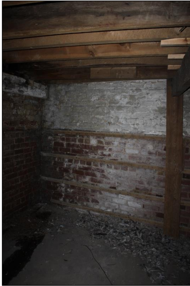
Figure 16a: Room D – In Situ Batons for Supporting Timber Panels
