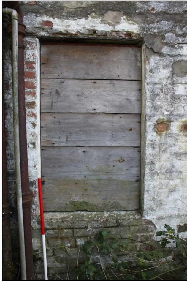
Figure 10a: Modern Window Inserted into W Elevation of Element 2 at Ground Floor Level
