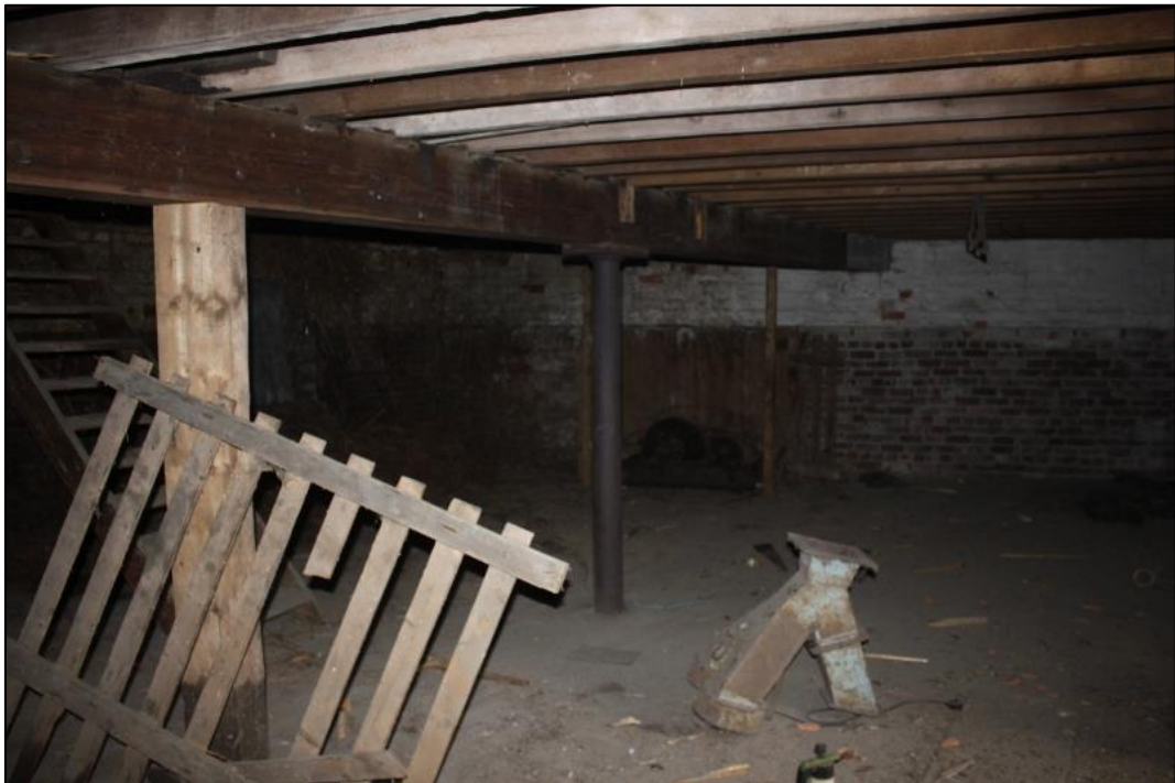
Figure 16b: Interior of Room E, Showing Central Beam and Supports
