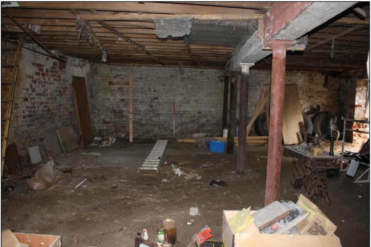
Figure 12b: Room C, Showing Central Timber Beam and Cast Iron Columns
