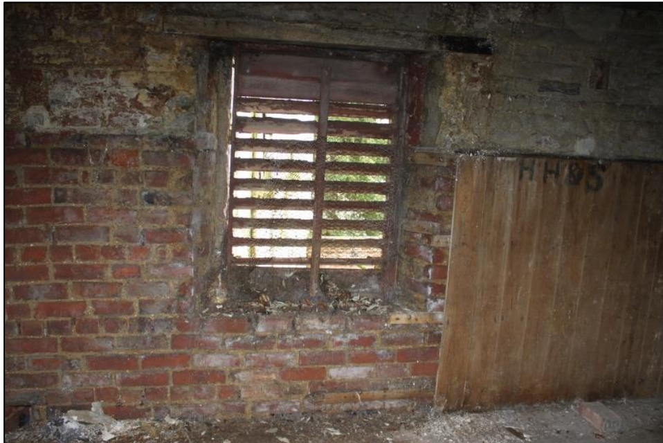
Figure 15a: Room D, W Wall, S End, Louvred Opening and In Situ Timber Panelling
