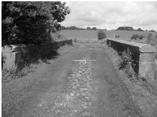
Fig. 6b: Mains Farm Bridge - Surviving Remnants of Cobbled Surface
