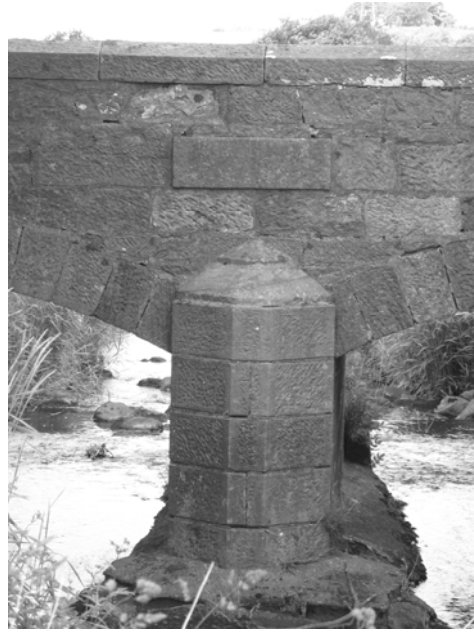
Fig. 7b: Mains Farm Bridge – Cutwater and Blank Datestone
