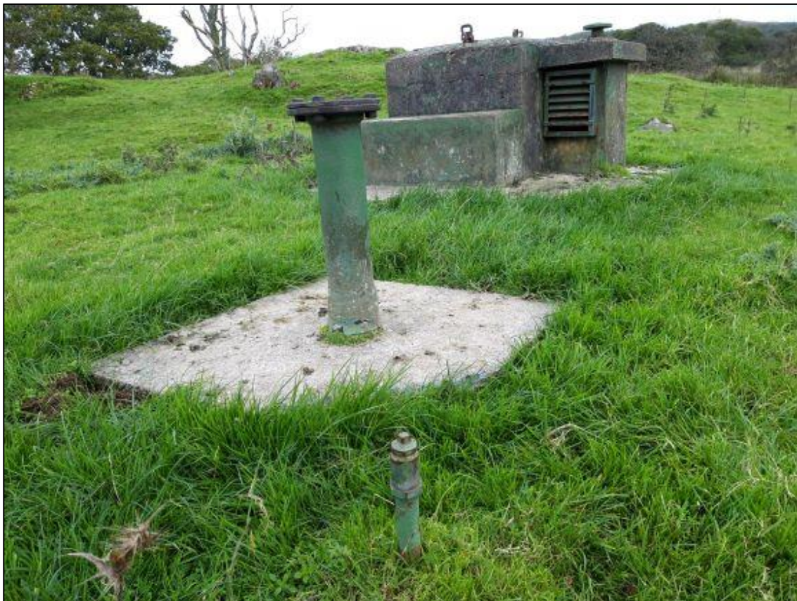
Figure 5b: Pipe (in foreground) possibly for a bomb power indicator baffle plate at S9
