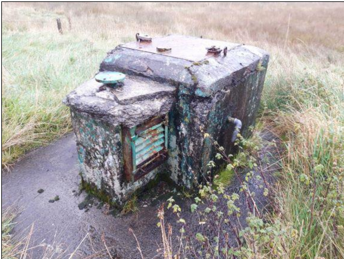
Figure 4b: Access Hatch at S7
