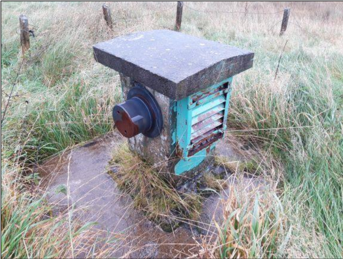
Figure 4a: Air vent at S7 showing the circular black cover attached to its side
