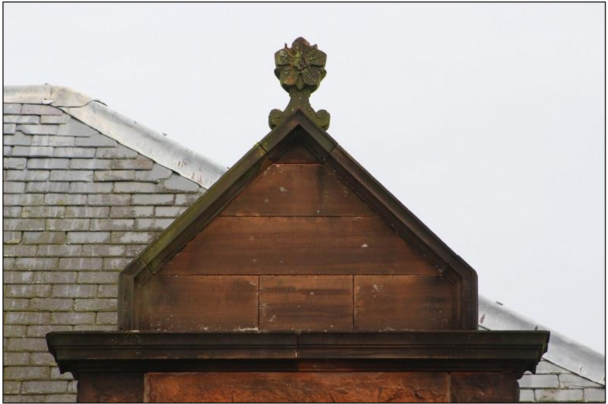
Figure 11a: Occupational Health Building – W Elevation, Detail of Pointed Pedimented Gablet with Rose Finial
