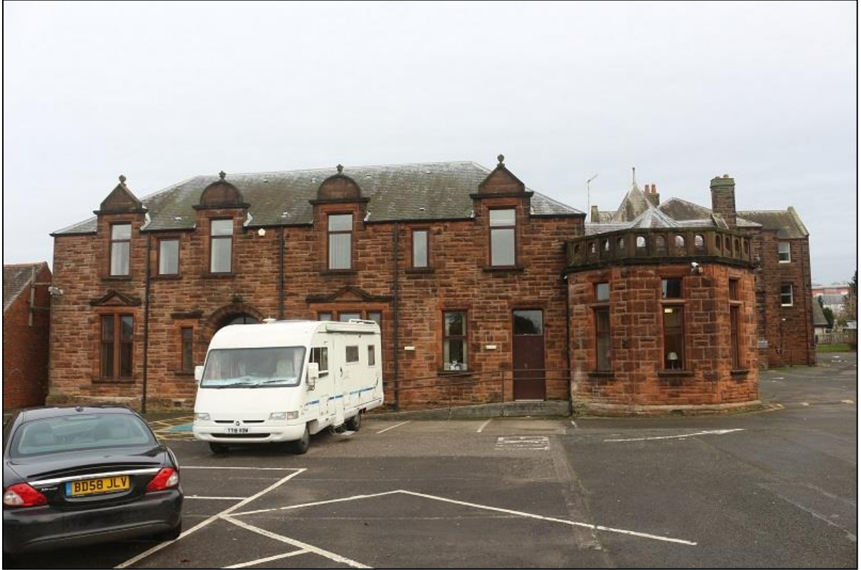
Figure 10a: Occupational Health Building – Principal (W) Elevation
