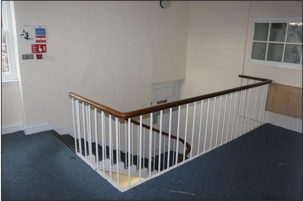
Figure 21a: Social Care Building – Stair at Second Floor Level
