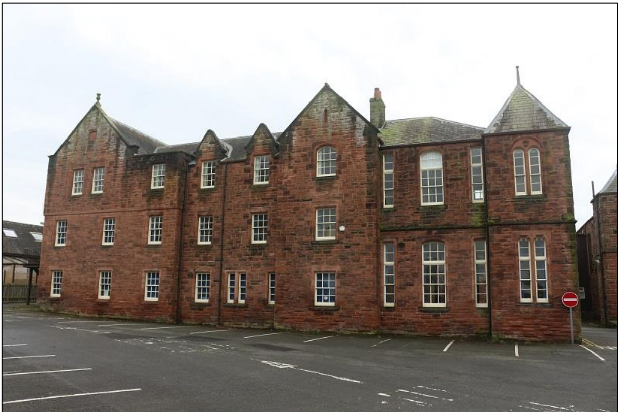
Figure 19b: Social Care Building – North Elevation, General View
