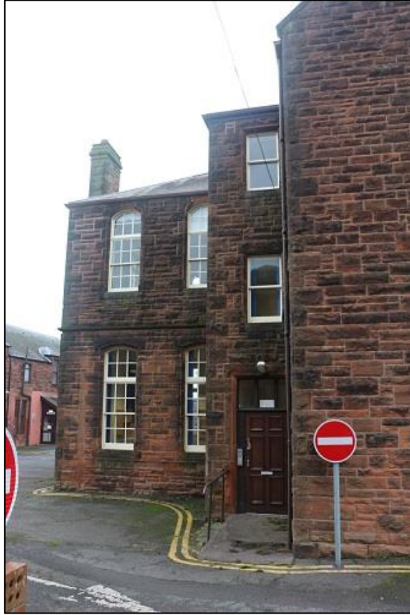
Figure 18a: Social Care Building – Main Entrance in S Elevation
