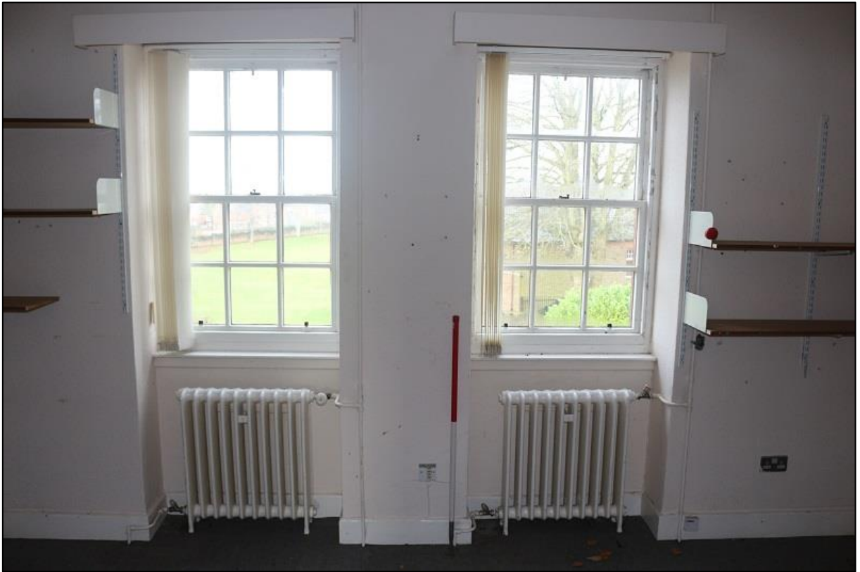
Figure 22a: Social Care Building – Windows
