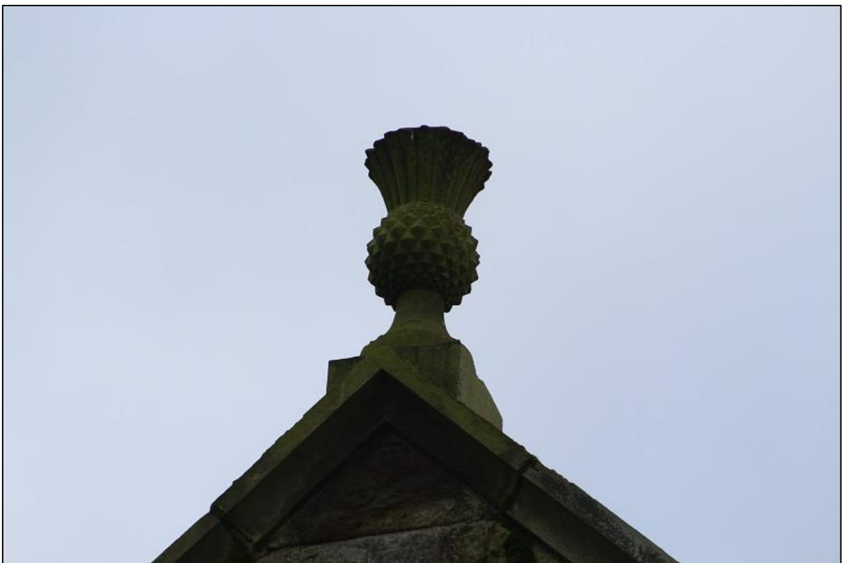
Figure 20b: Social Care Building – Thistle Finial Surmounting Gable at E End of N Elevation
