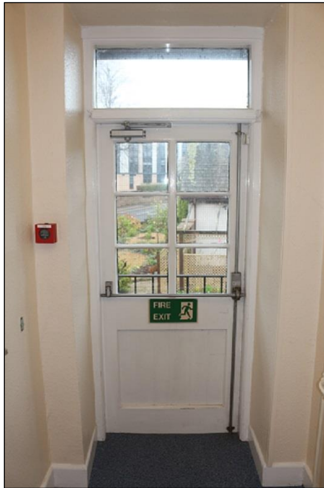
Figure 21b: Social Care Building – Door Onto Fire Escape, 2 nd Floor Level
