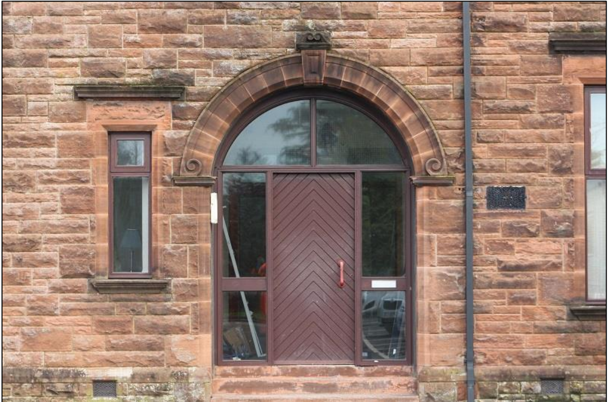
Figure 10b: Occupational Health Building – Main Entrance in W Elevation
