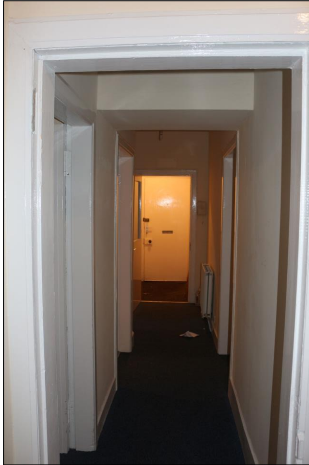
Figure 7a: North Lodge, Looking S from Rear of Property Through Room NL2 (Corridor) to Room NL1 (vestibule)
