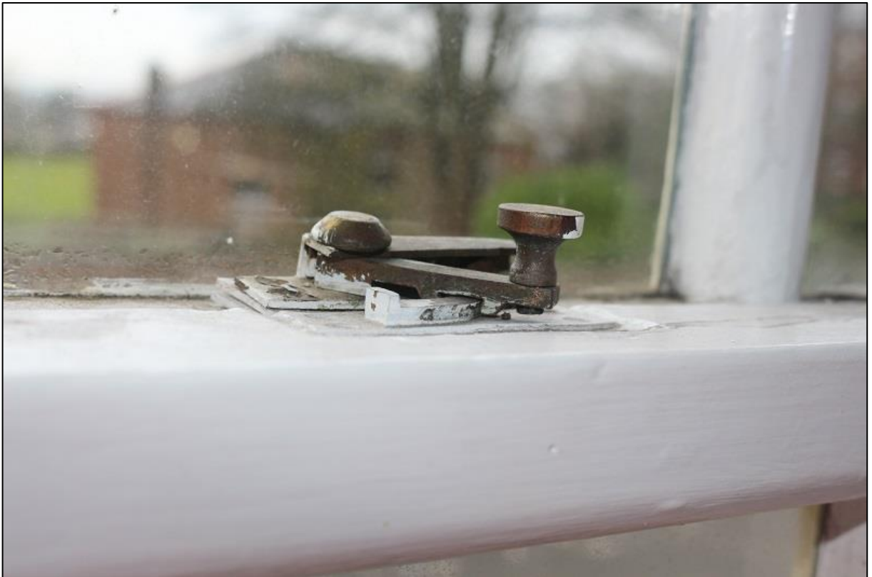
Figure 22b: Social Care Building – Example of Original Window Latch
