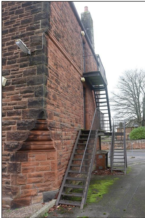
Figure 18b: Social Care Building – External Fire Escape on E Elevation
