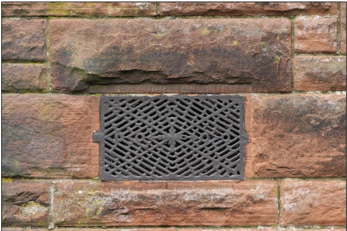
Figure 13b: Occupational Health Building – Cast Iron Ventilator Grille, W Elevation
