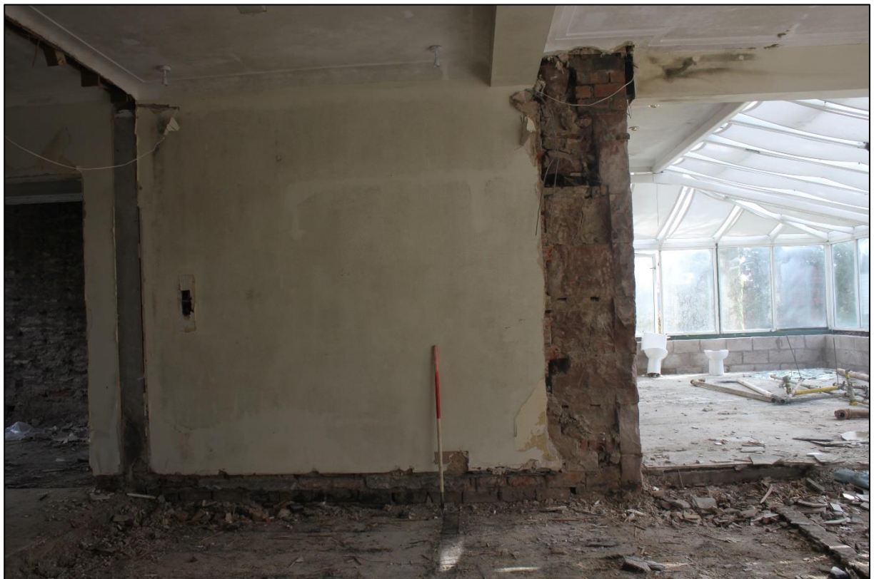
Figure 14a: SE Wing (Late 19 th Century) – Room a, Former Window in SW Wall
