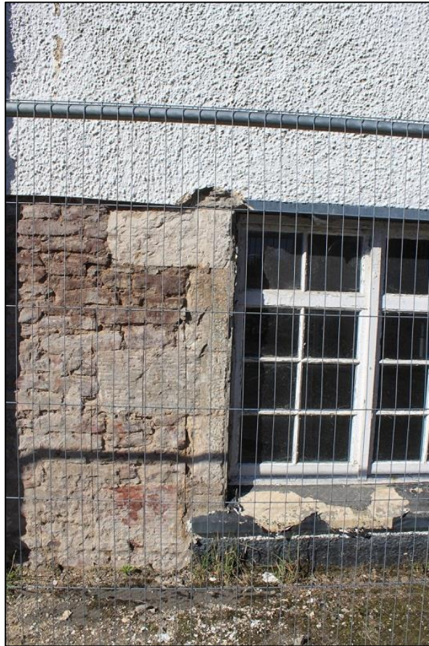
Figure 11a: Relict Margin and Sill at SE End of Window in NE Elevation (Exterior, Room q)
