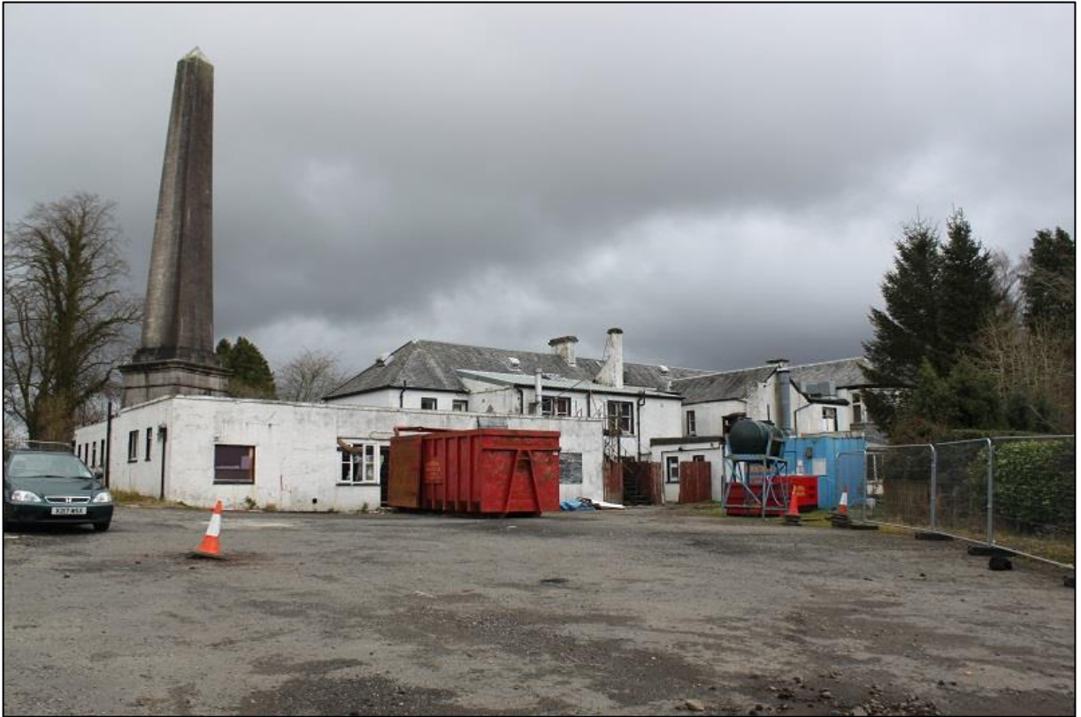
Figure 16a: View of Rear, SW, Elevation, Showing Later Extensions and Additions
