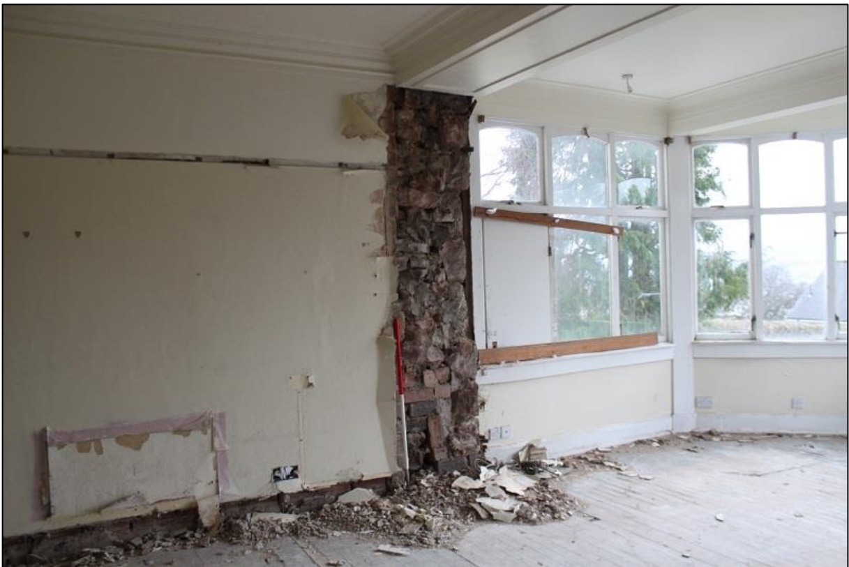
Figure 17a: Interior Room 1d, Showing Later Extension Abutting Late 19 th Century Fabric
