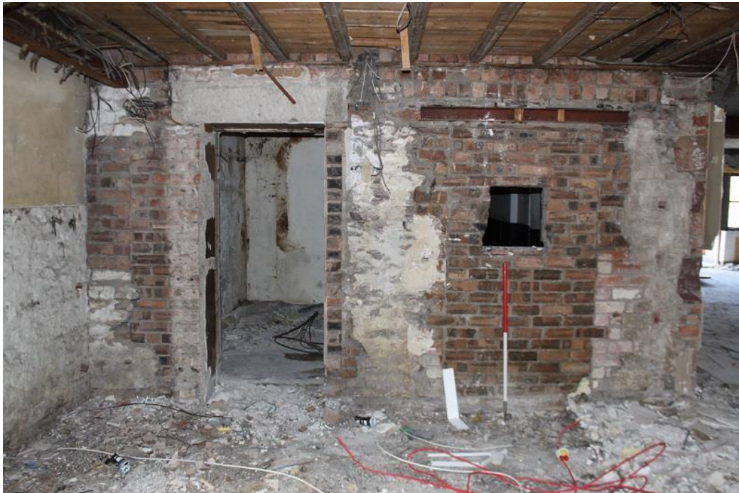
Figure 9a: Room q, blocked window and raised wallhead, NW end NE Wall
