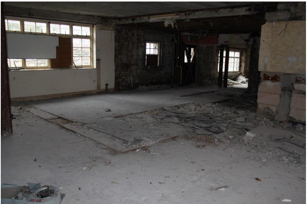
Figure 16b: Interior Room r, looking S Towards Historic Core of Building
