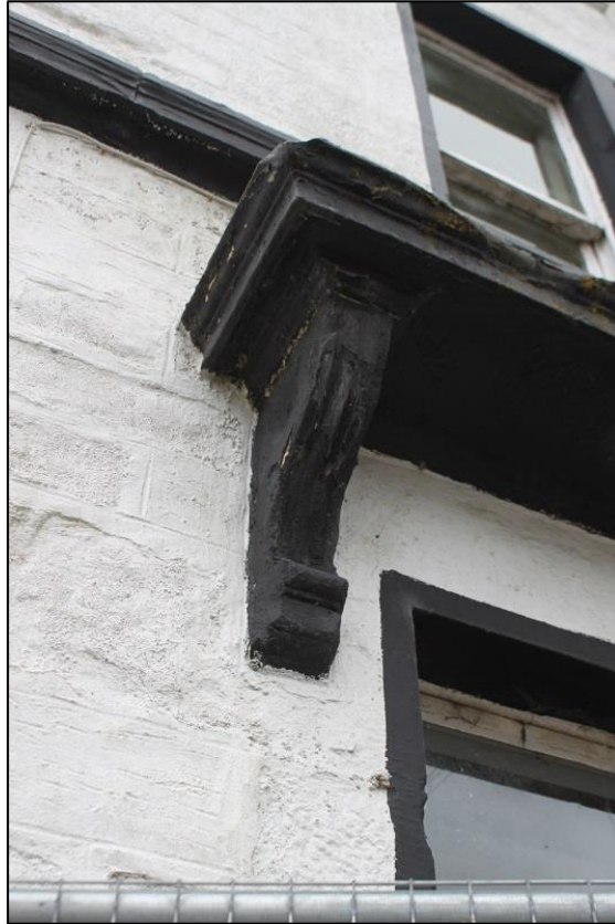
Figure 12a: SE Wing (Phase 2, Late 19 th Century) – Corbels Supporting Projecting Cornice Moulding
