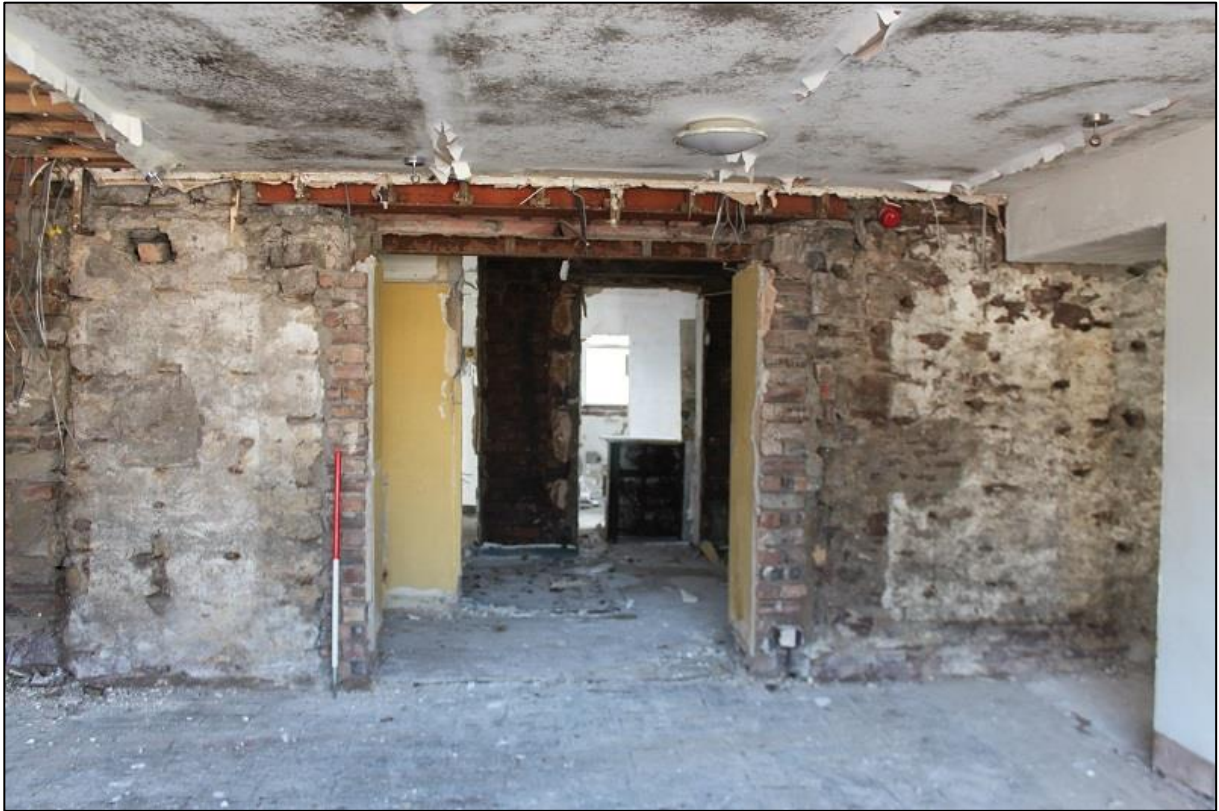
Figure 7a: Roof j, Opening at NW End of SW Wall
