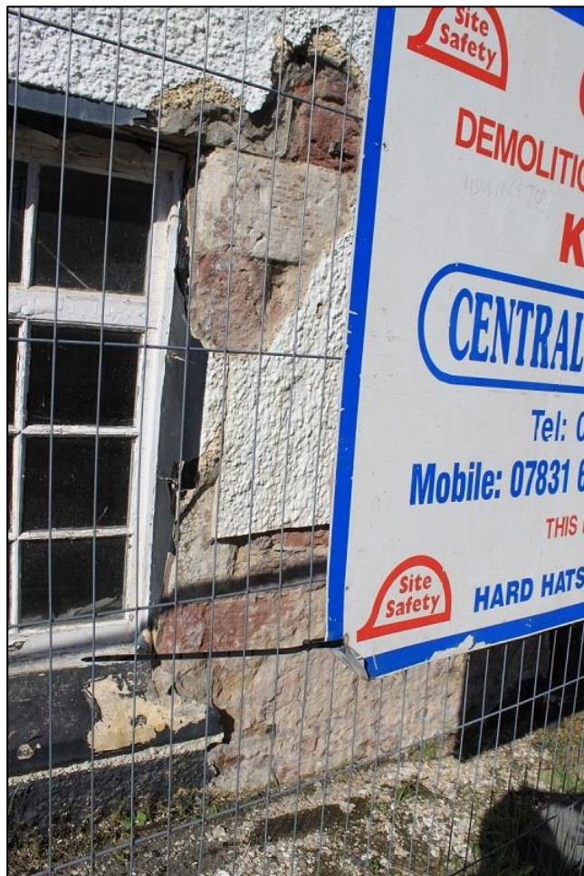
Figure 10b: Relict Margin of Blocked Window, NW end Extant Window in NE Elevation (Exterior, Room q)
