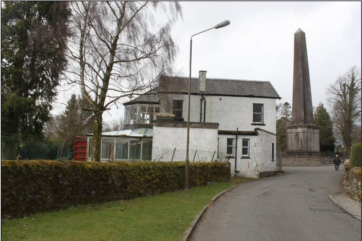
Figure 17a: SE Elevation, Showing Late 19 th century Wing With Later Additions to Rear
