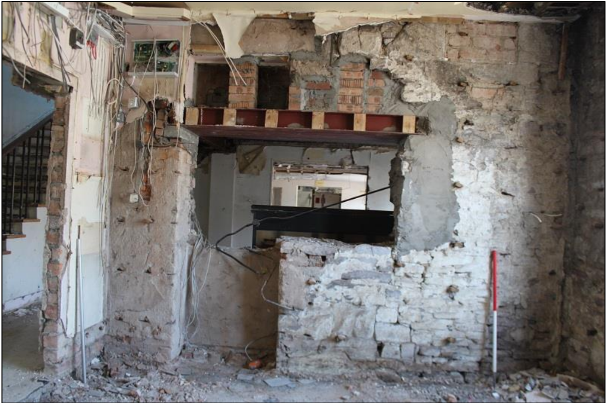
Figure 5a: NW Wall of Room g, Showing Surviving Early fabric at NE Side & Basal Levels
