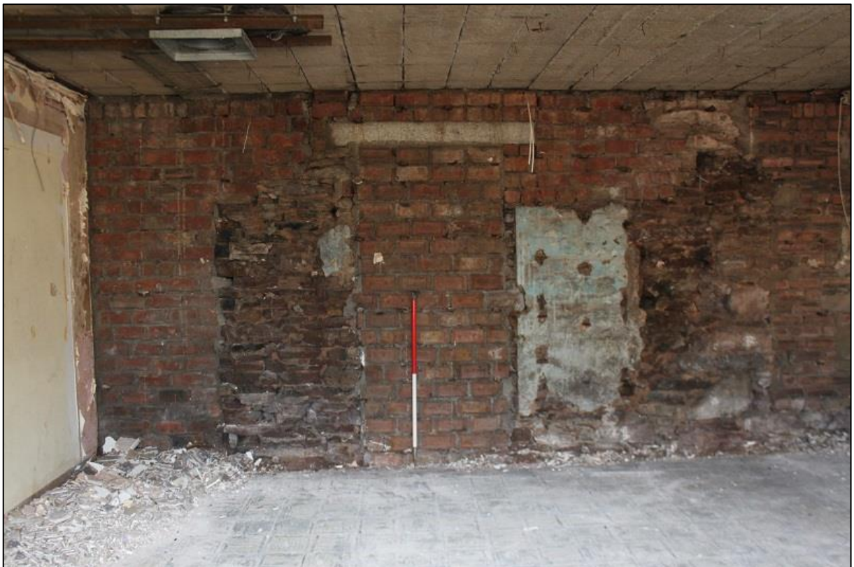
Figure 6b: Room j, Rear SW Wall
