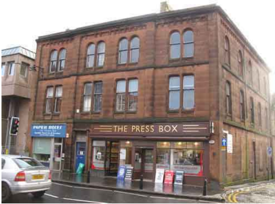
Figure 2a: 100-106 John Finnie Street, W-Facing Elevation
