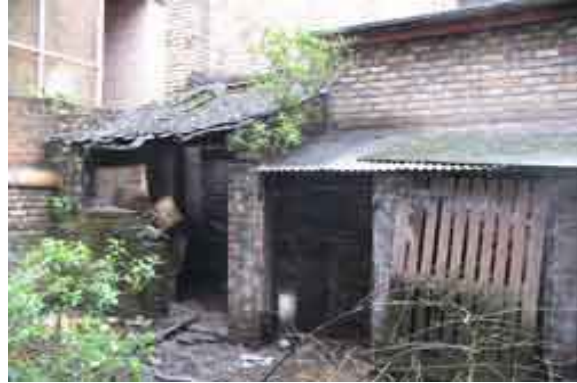
Figure 4b: Wash-house, Outbuilding & Perimeter Wall
