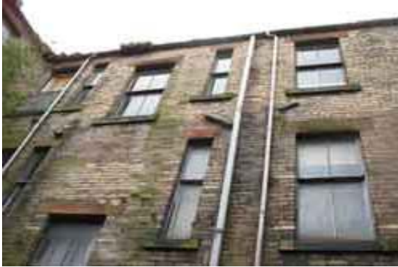
Figure 4a: Exterior, E-Facing Elevation
