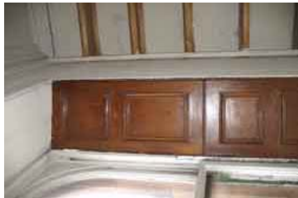
Figure 5f: In Situ Timber Panelling, Room 104. Flat 1
