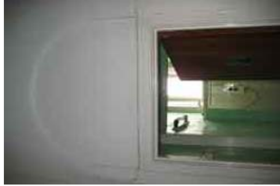
Figure 5a: Infilled Arched Entrance, Flat 5 (1st Floor)
