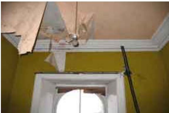
Figure 5e: In Situ Cornice, Room 213 (Flat 2)
