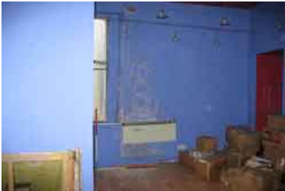
Figure 5c: Former Kitchen/WC Area 101 (Flat 6)
