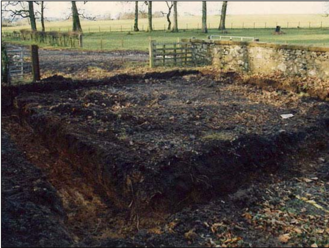
Figure 4a: Foundations of garage excavated
