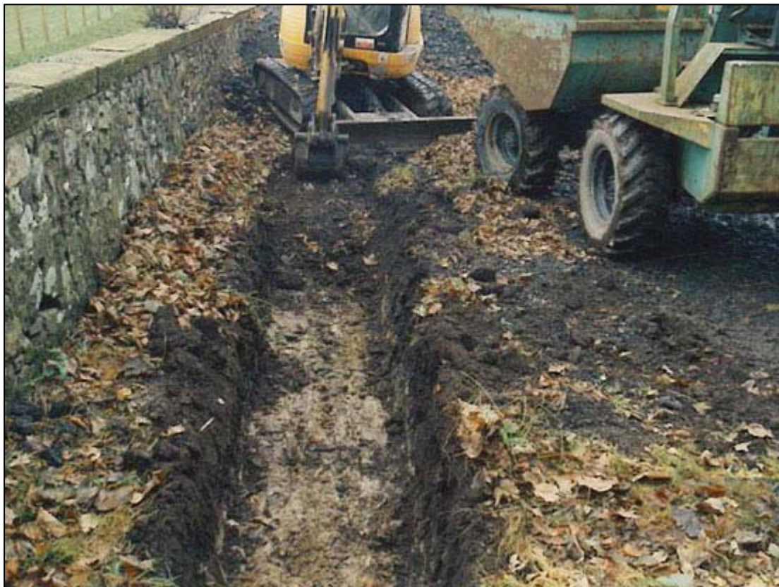
Figure 3b: Excavation of the garage foundations
