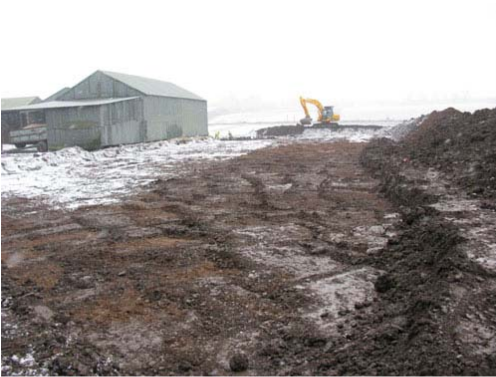
Figure 1a: Site after monitored strip.
