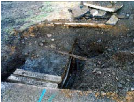
Figure 3e: Test Pit 5
