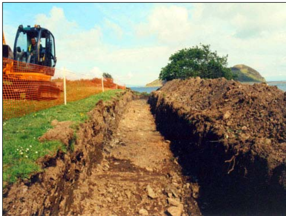
Figure 4b: Pipe Trench
