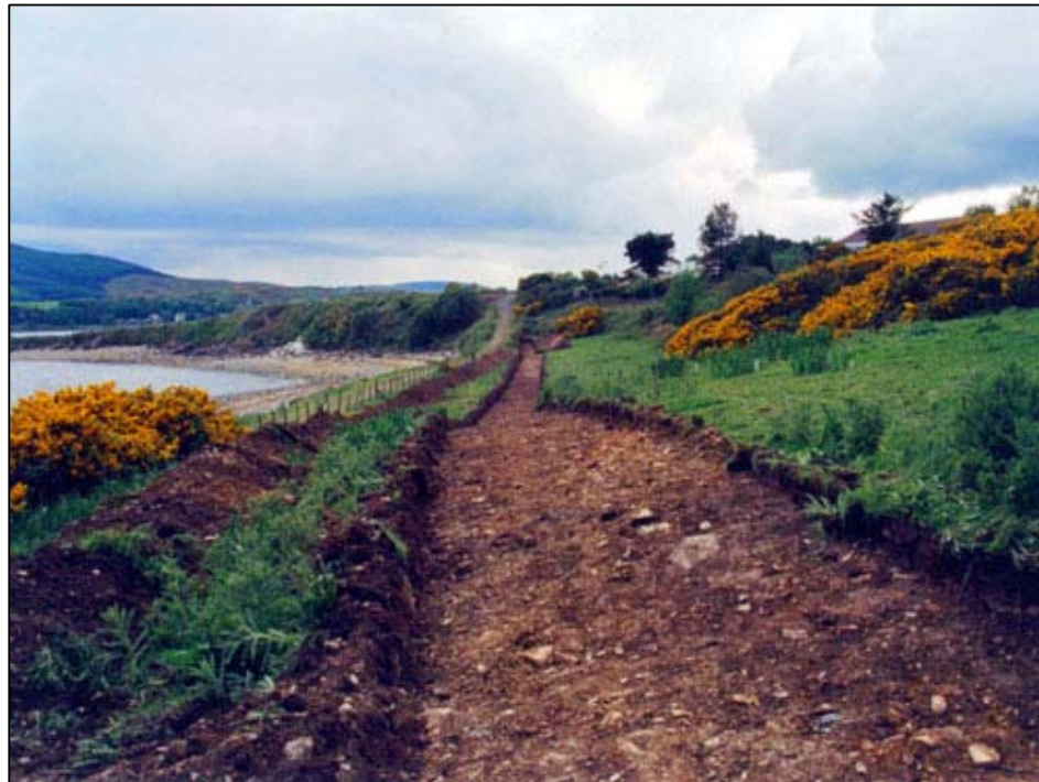
Figure 4a: Beginning of the pipe trench looking to Trench Point
