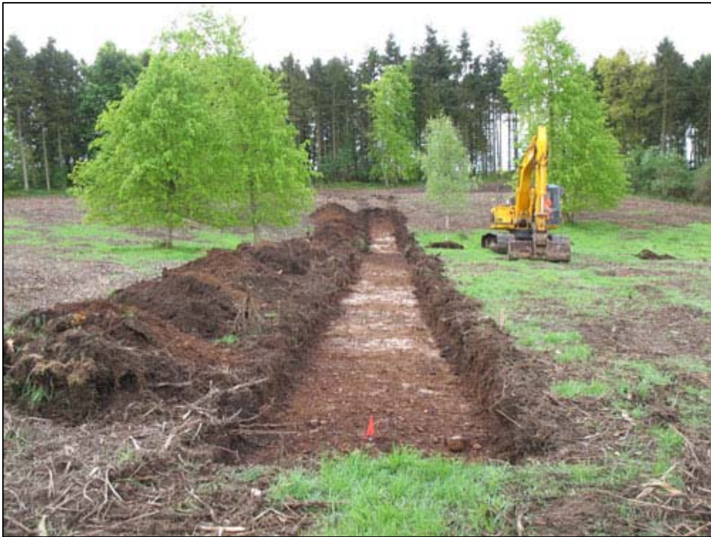
Figure 3a: Trench 10 looking south
