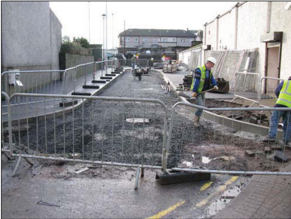
Figure 3a: Area1: Work in Progress
