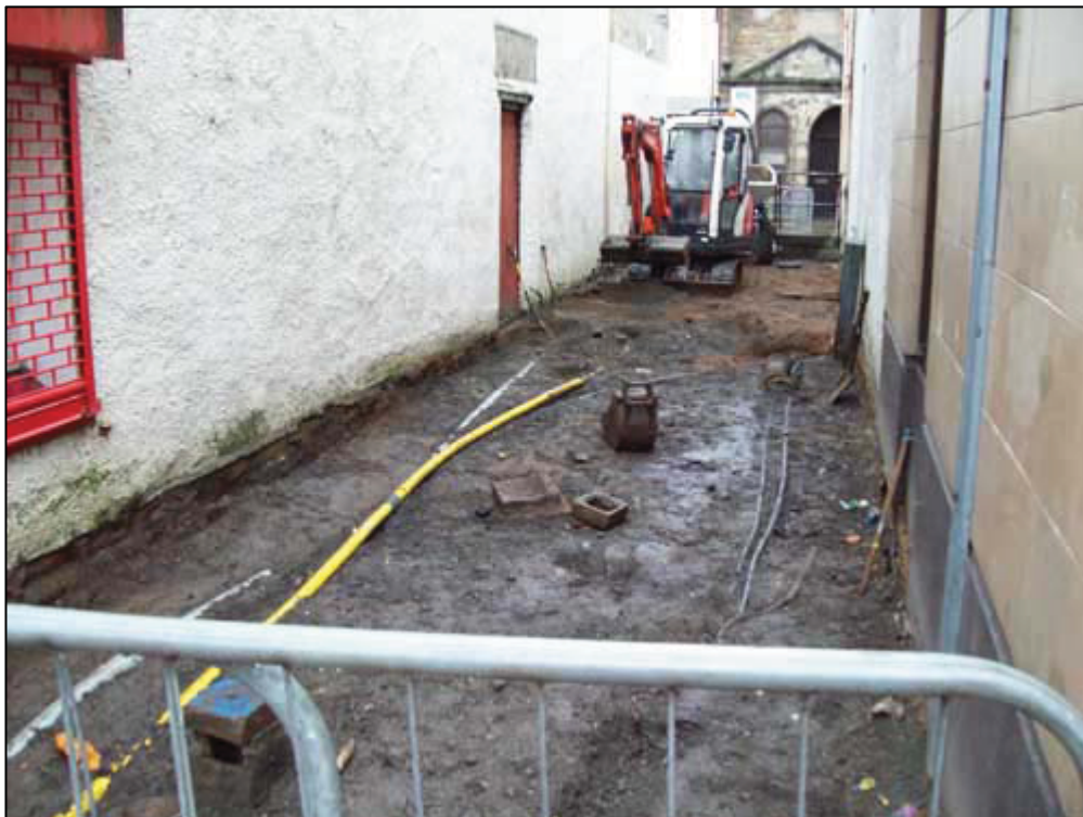
Figure 10b: Area 7: Ground Reduction Completed
