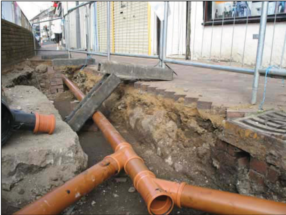
Figure 12b: Wall (018), to W of Area 2
