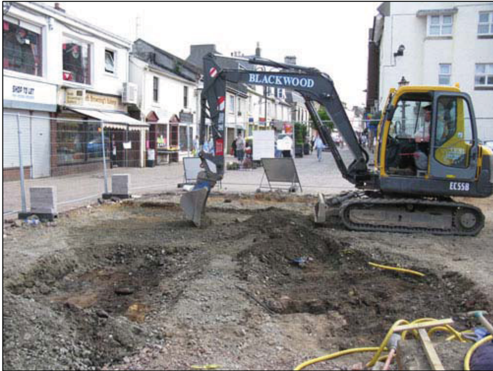
Figure 4a: Area 2: Ground Reduction in Progress
