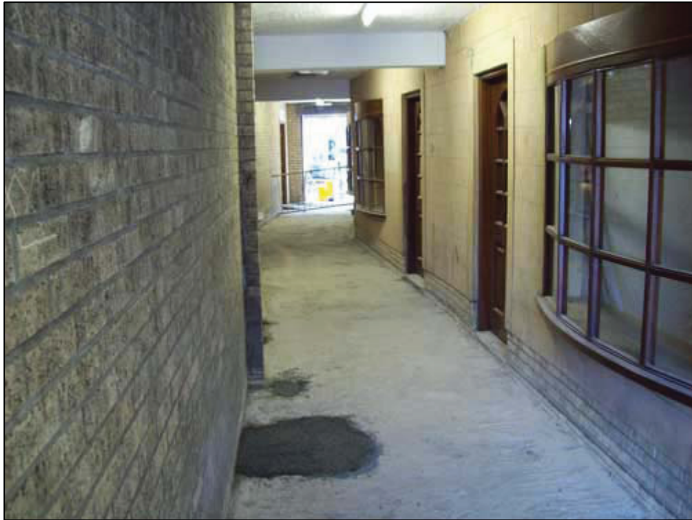
Figure 11a: Area 8: Work in Progress
