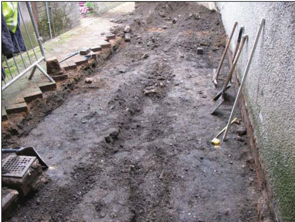
Figure 11b: Area 9: Ground Reduction in Progress
