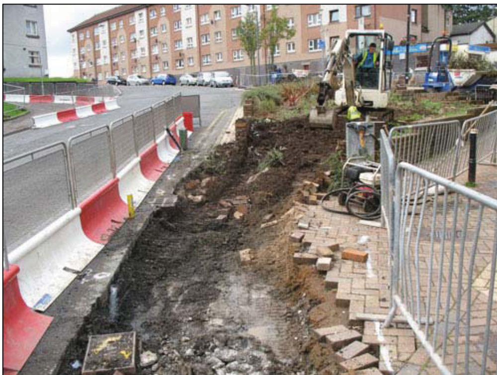
Figure 8b: Area 4: Initial works – Removal of Extant Flowerbed
