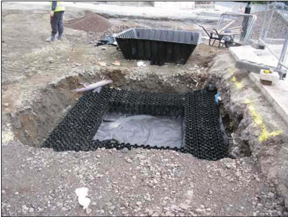
Figure 8a: Excavation of Tree Pits in Progress
