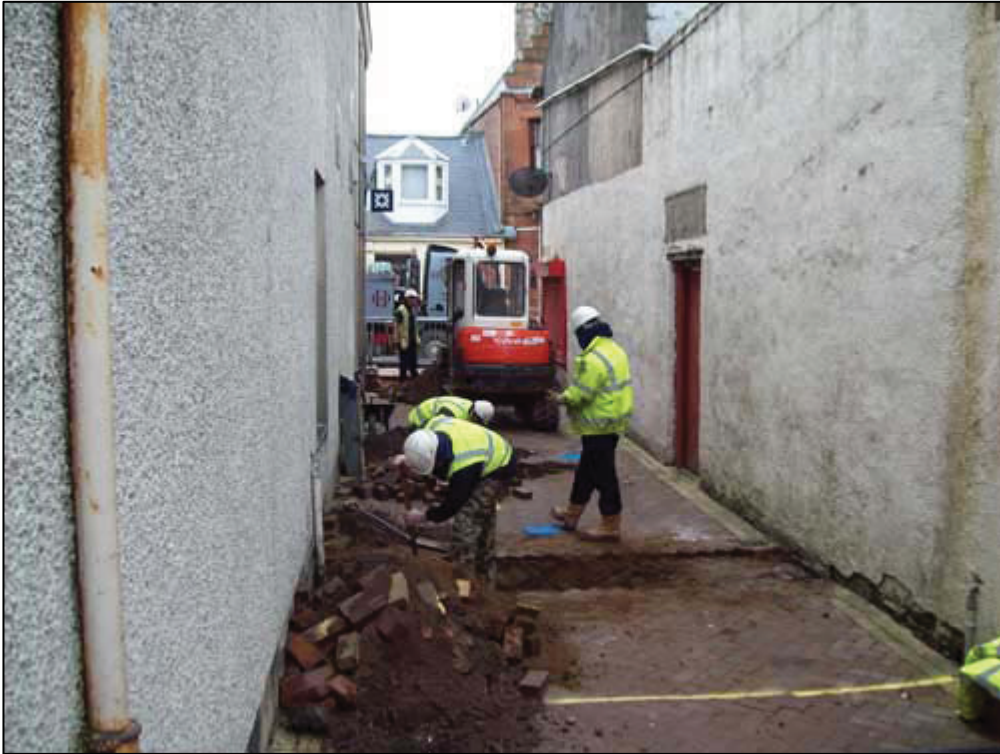
Figure 10a: Area 7: Initial Works
