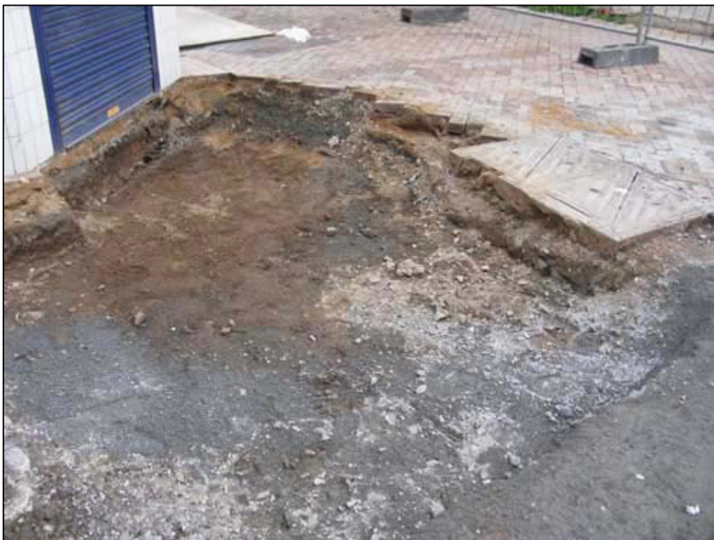
Figure 9b: Area 6: Works Commencing
