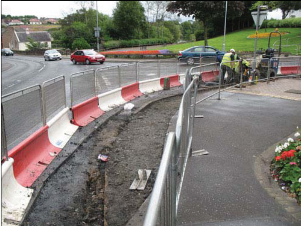
Figure 9a: Area 4: Works Continuing to N (Lachlan Way)
