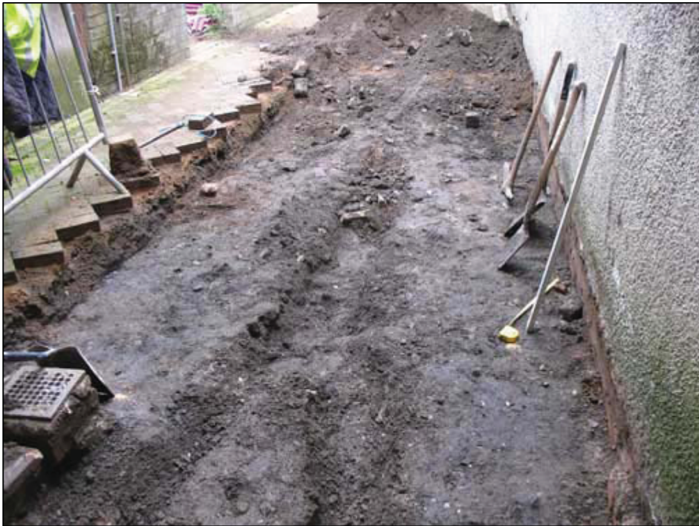
Figure 12a: Area 10: Ground Reduction in Progress
