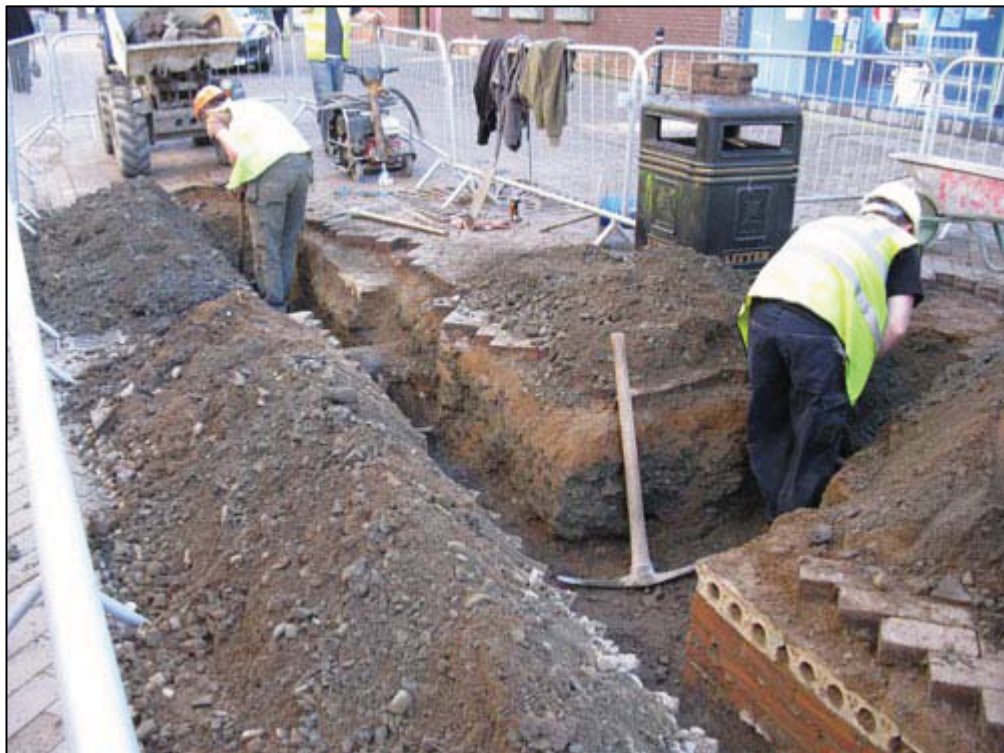
Figure 4b: Area 2: Excavation of Service Trench
