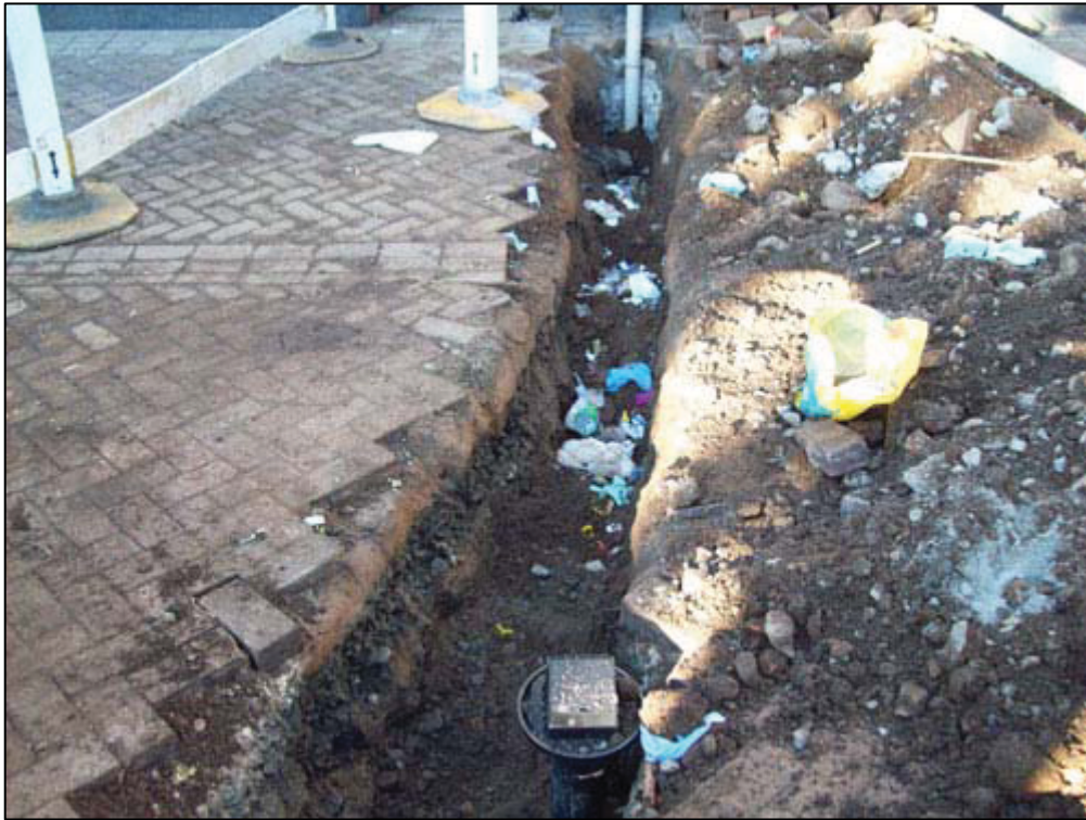
Figure 5a: Area 3: Initial Excavation for Services
