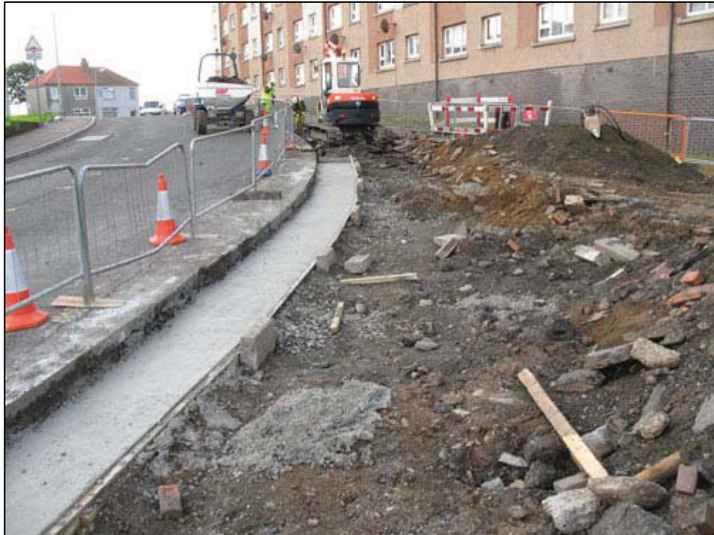
Figure 7b: Area 4: Work in Progress
