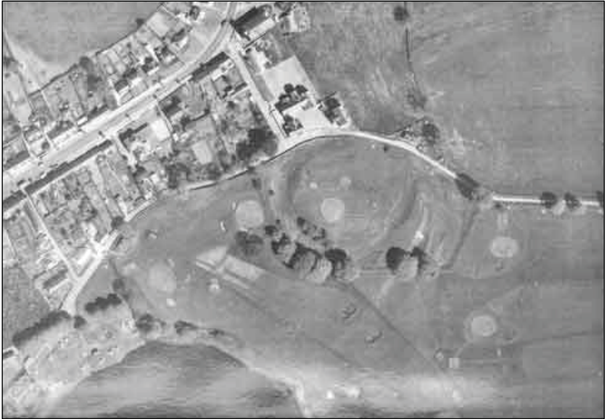
Fig. 3a: Vertical aerial photograph showing Lochmaben Motte prior to enlargement and build up of tees, etc. (c.1948)
