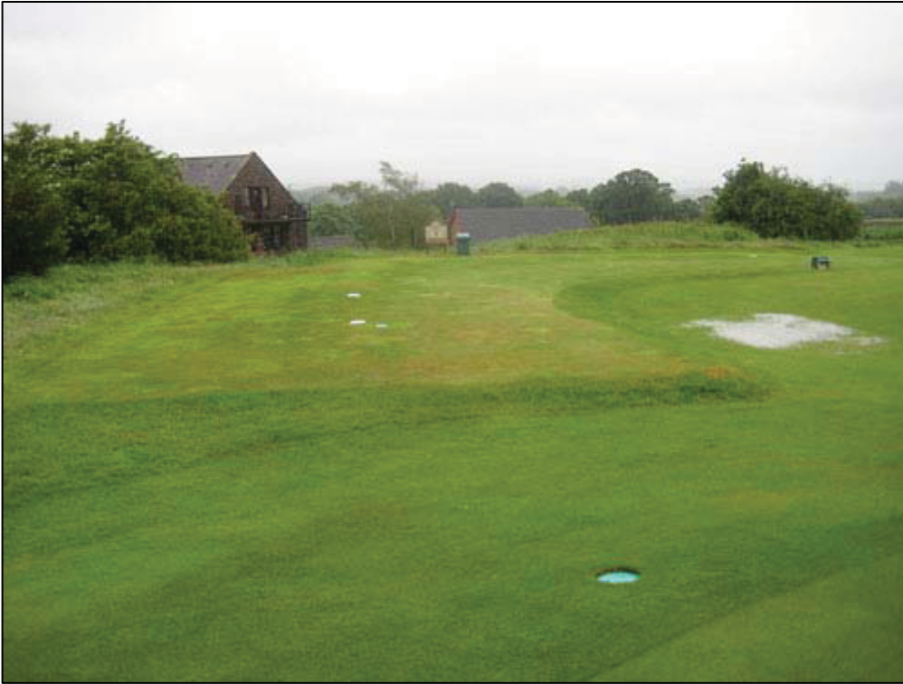
Fig. 4a: Main Tee for 3rd hole on the summit area (from north edge 2nd Green), note standing water to front of raised tee
