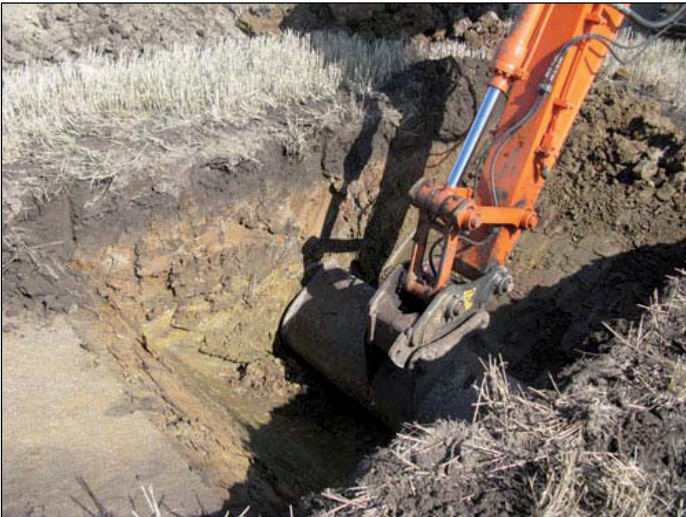
Figure 4b: Test pit to test subsoil – Trench 27
