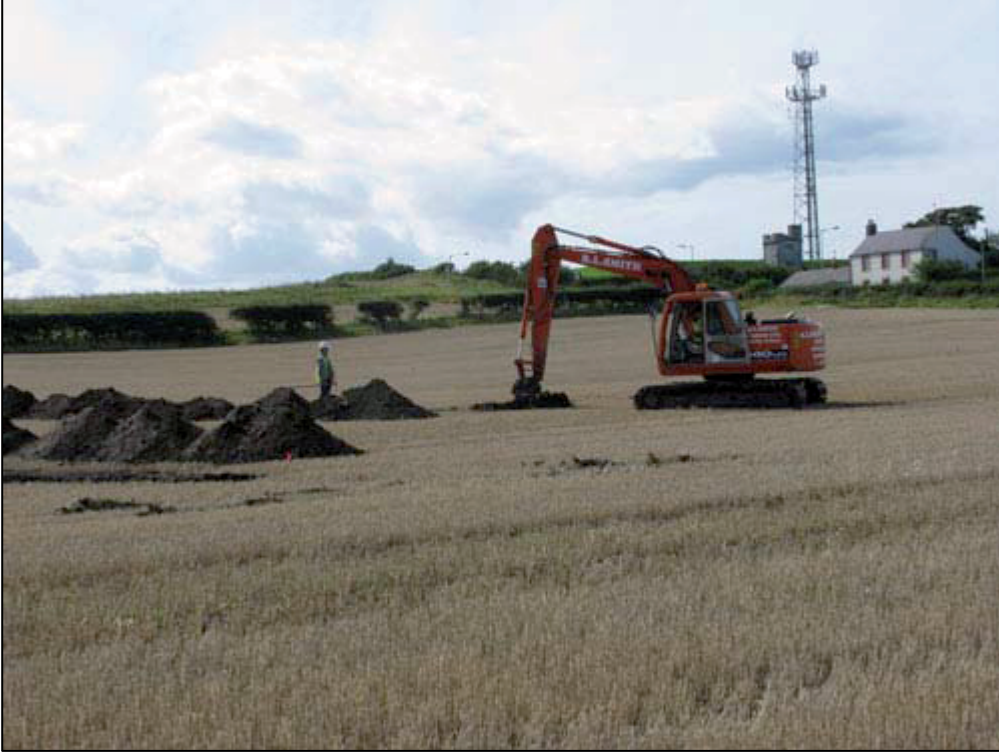
Figure 2a: Working in the north field.
