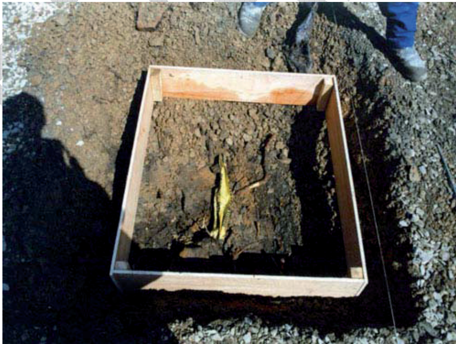
Figure 3b: Pad 5 with top of gas service trench
