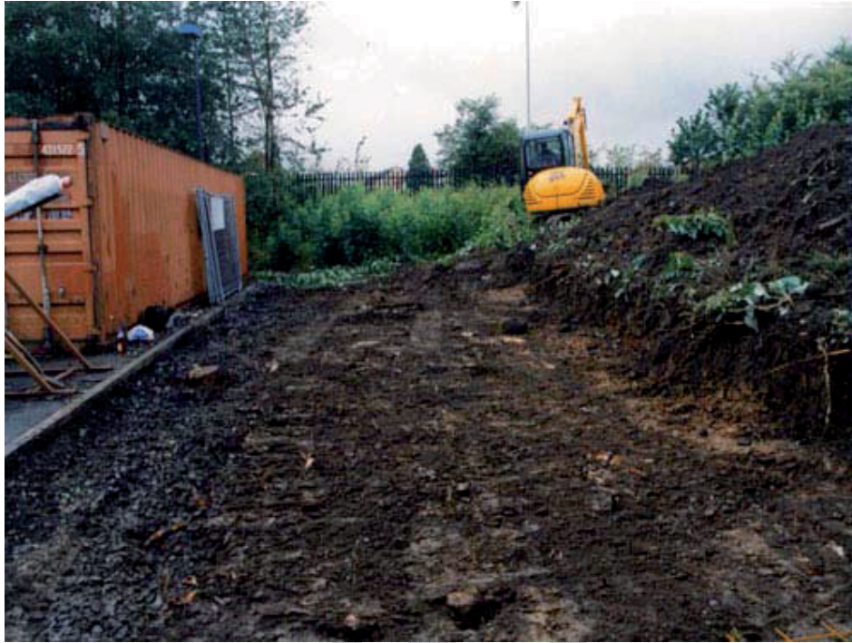
Figure 3a: Levelled Area
