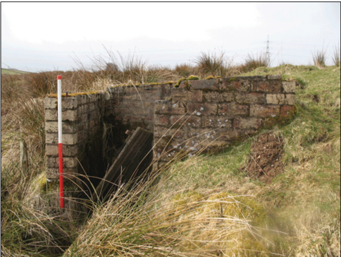
Figure 8b: Pump S5
